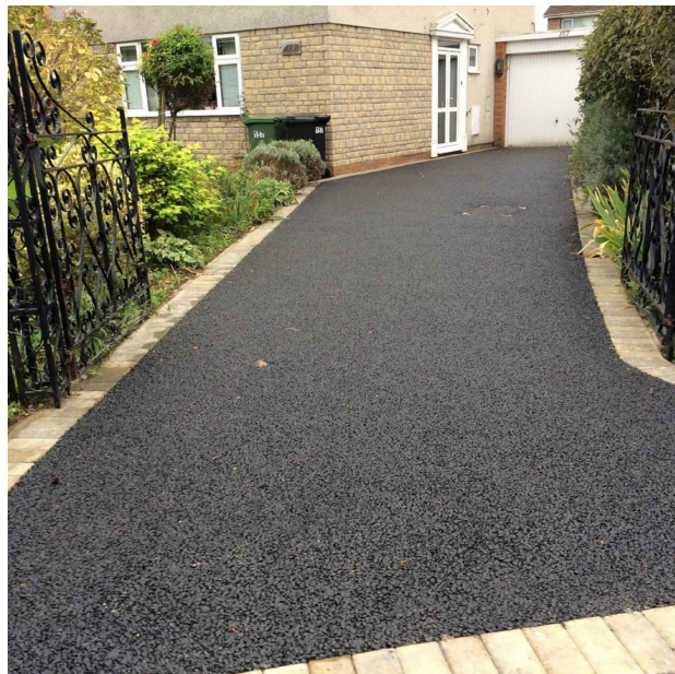
M3 - TARMAC ROAD AND PARKING AREAS
