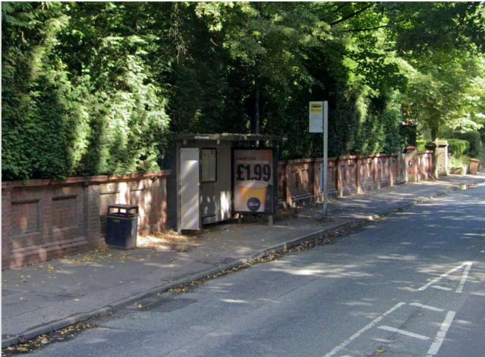
Northbound view of existing shelter
