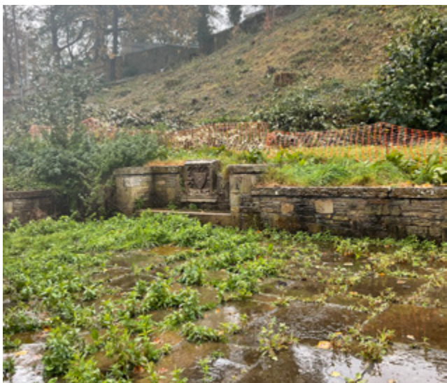
3.56 Retaining wall with the Borough coat of arms
