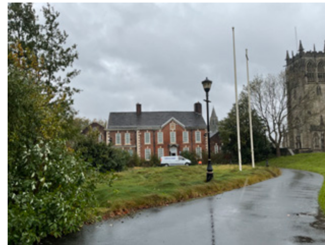
3.24 Old Vicarage, viewed from the south
