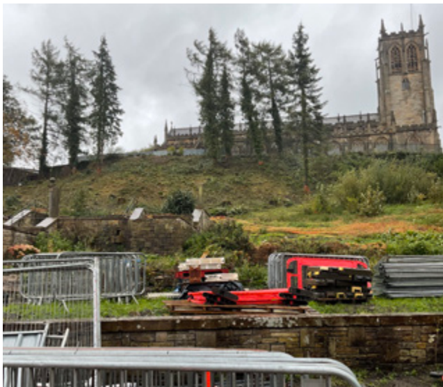
3.43 North boundary wall to Packer Spout Gardens, matching the walls of the centrepiece
