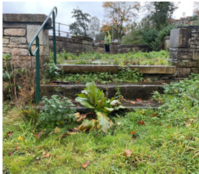
3.63 Modern inserted opening, steps and handrail
