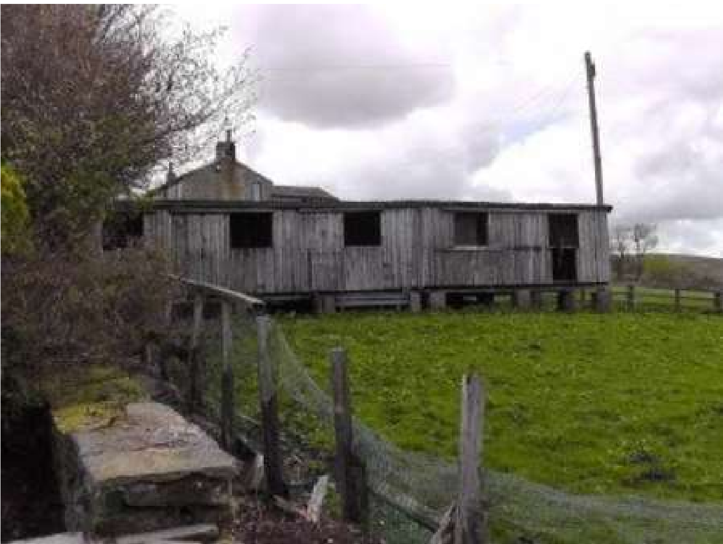
One of the buildings removed and returned to grass:
