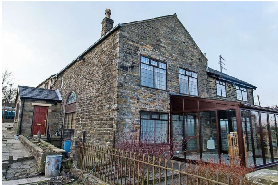
House before work:
