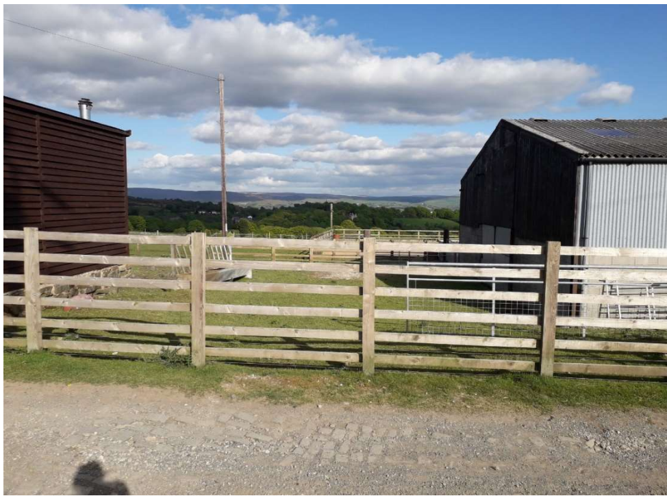
Photo from Bridle Way looking down the field between the barn belonging to Knacks Farm and the boundary edge of 4 The Knacks. The current arena is partially obscured from view by 2 lines of fencing which are both between the Bridle Way and the arena fence, the same would apply to an extended arena.
