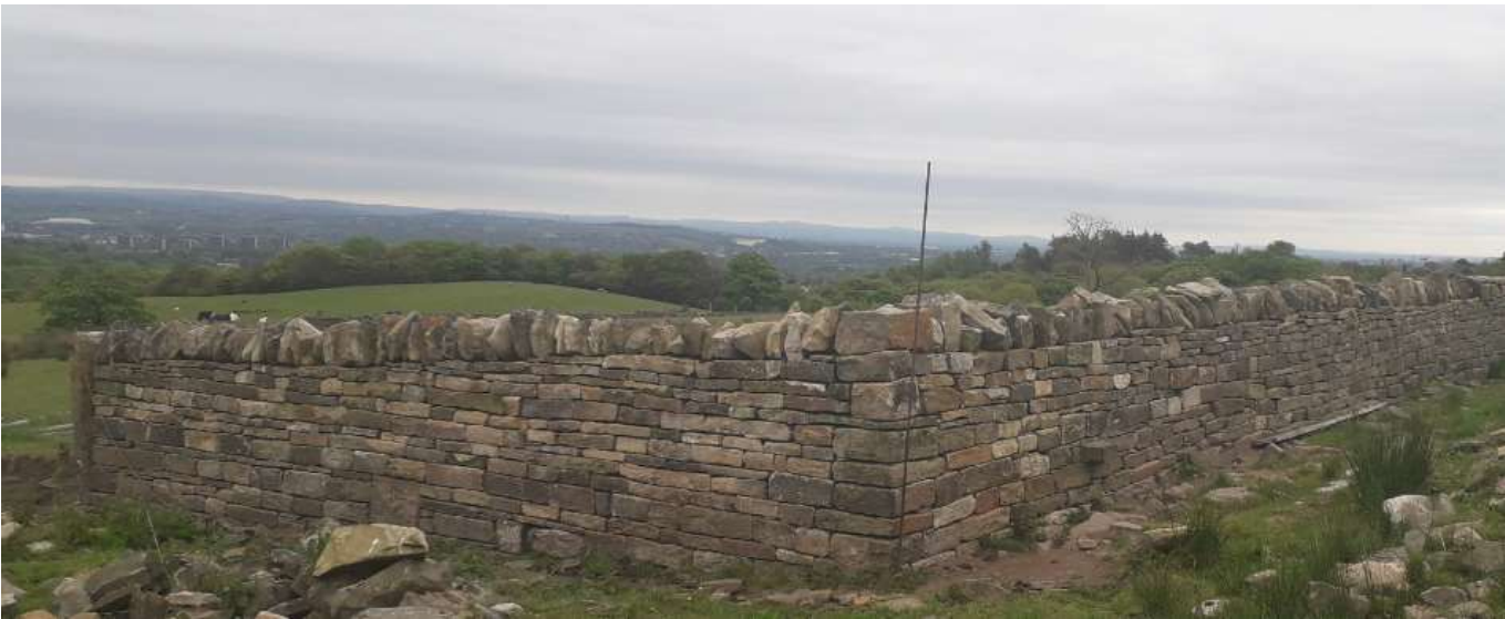
Walls / fences after work:
