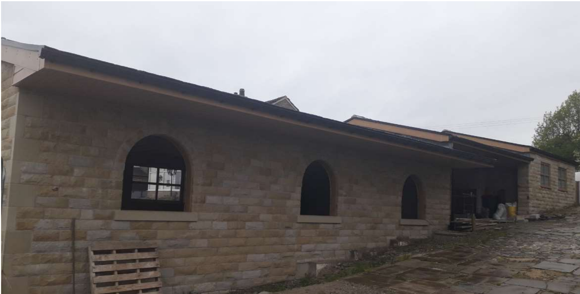
Outbuilding after work:
