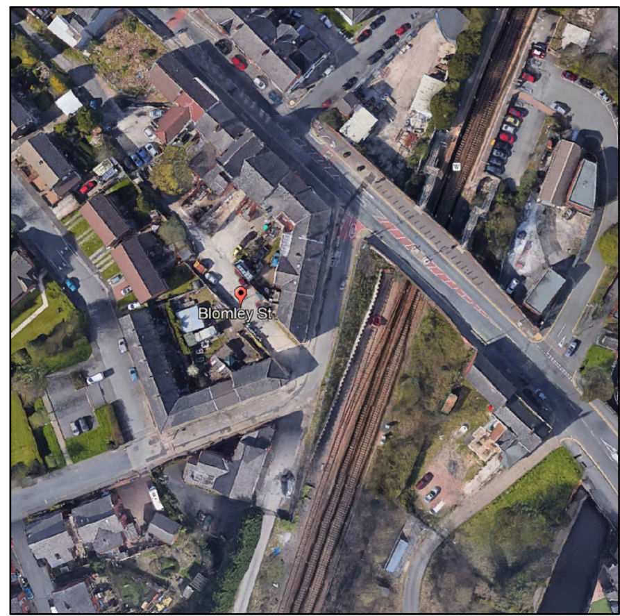
NORTH SOUTH AERIAL VIEW
