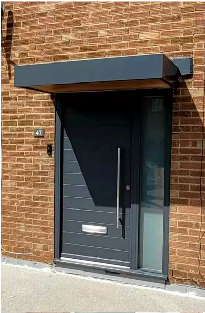
6 Entrance Door Canopies Colours: RAL 5014, 6033, 6018 (to match corresponding door colour) Weathered finish to top with flashing at junction with Brickwork above.
