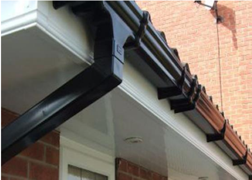
Black plastic Ogee gutters with matching square section downpipes to match gutters and downpipes serving main house.
