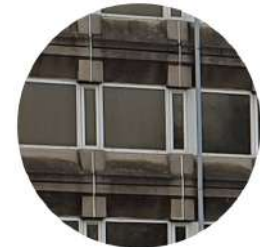
SQUARE REPETITIVE WHITE WINDOWS SANDWICHED BETWEEN CANTED CONCRETE RIBBONS
