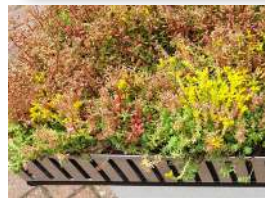
Green Roof Sedum Trays
