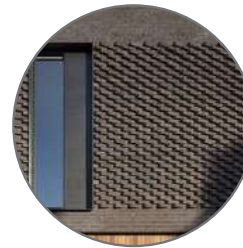
FEATURE BRICK BANDS & PATTERNS (20MM PROTRUSION) COLOURS - CHARCOAL, WHITE & GREY
