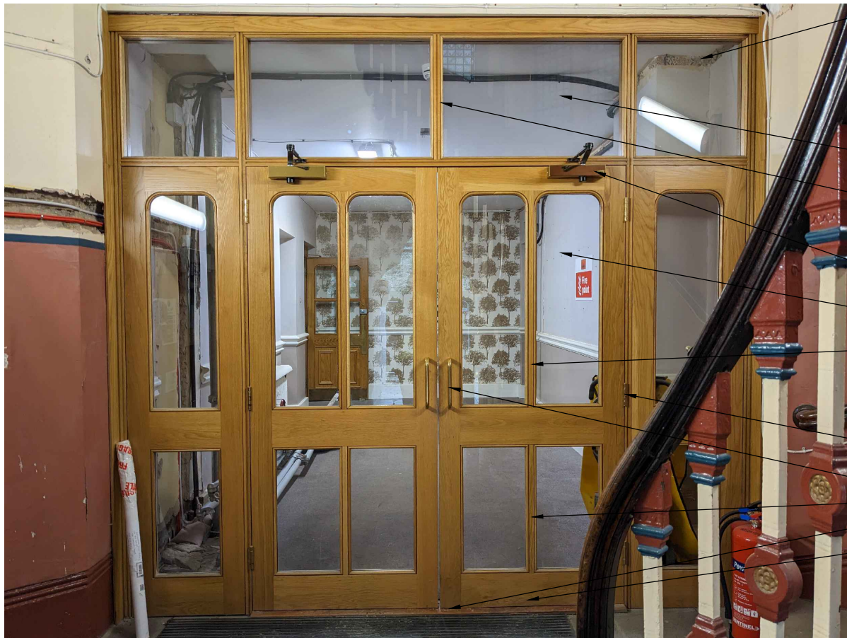
EXISTING VIEW OF DOOR FROM G12 (STAIR) SIDE
