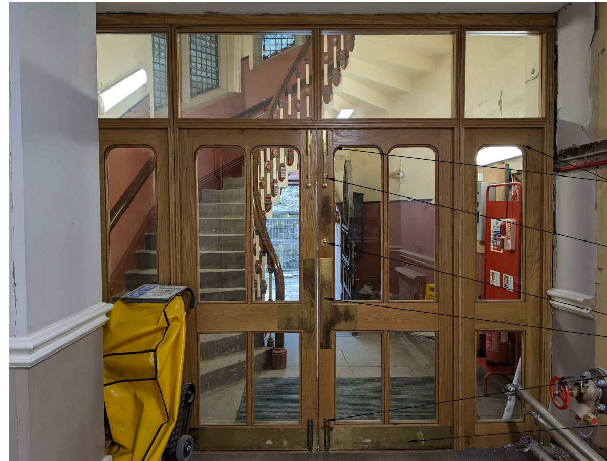
EXISTING VIEW OF DOOR FROM G13.a (STAIR) SIDE
