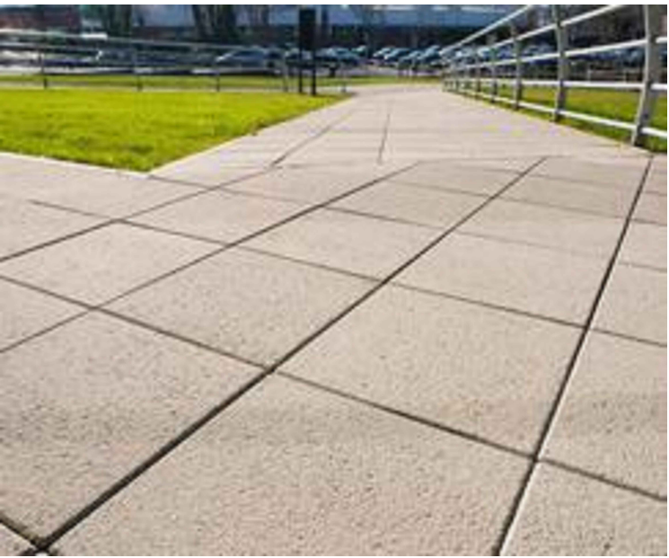
M2 - Buff flagged paths Buff 450 x 450mm flags on coarse sand & compacted ground
