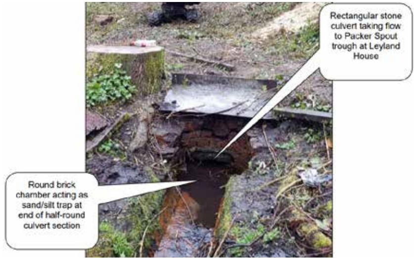
Sample of historic drainage identified alongside rill reinstatement
