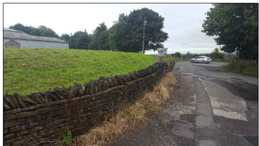
Image of the existing dry stone wall with vertical coping at the entrance to the site from Wildhouse Lane. The proposed wall is to match the vernacular of the existing wall.
