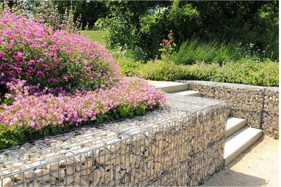
1M high gabion basket retaining walls
