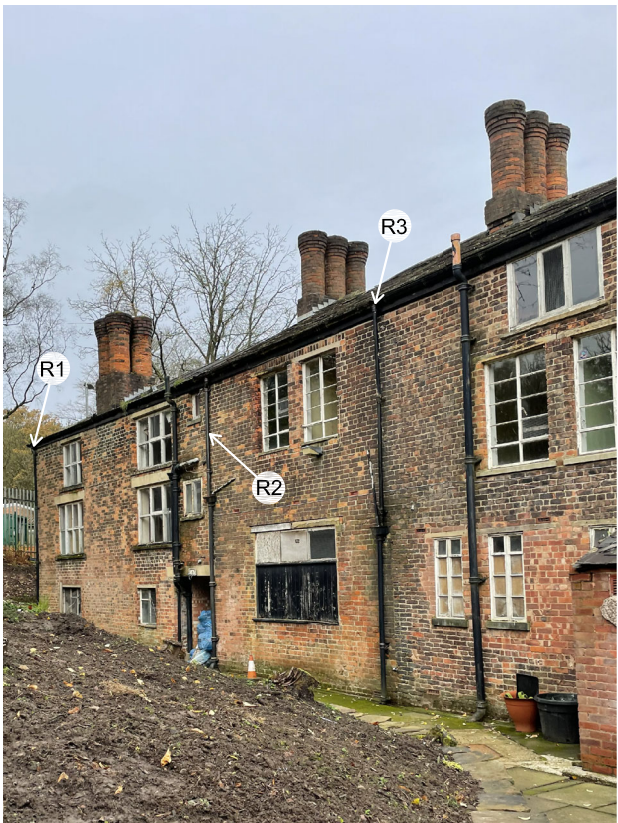
Site photos showing hoppers and down pipes
