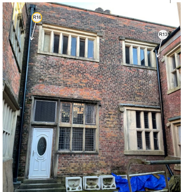
Site photos showing hoppers and down pipes
