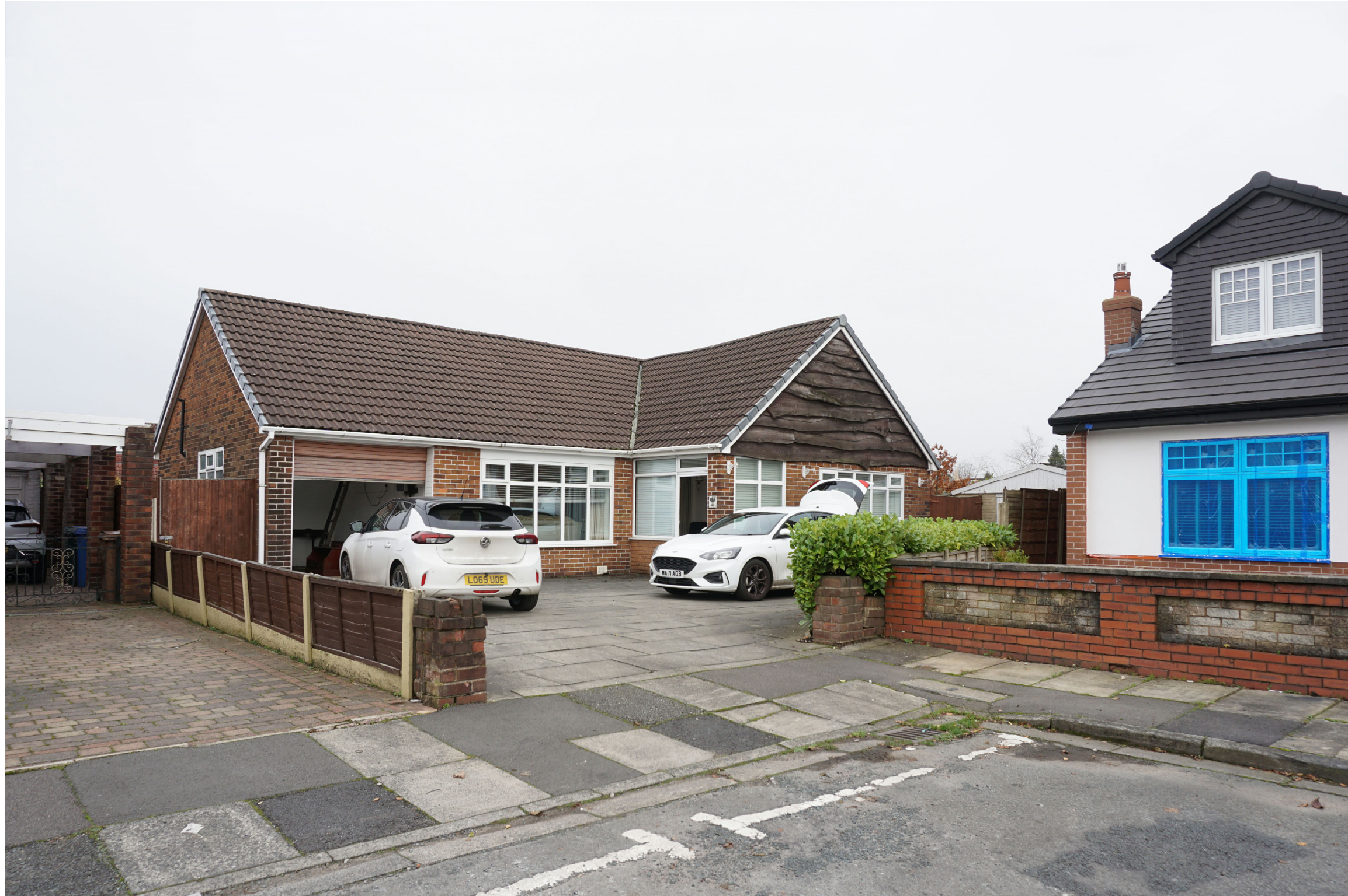
01 EXTERIOR VIEW FRONT - EXISTING NTS
