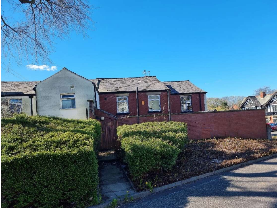
Rear Elevation - showing access to rear yard area, boundary wall and first floor windows
