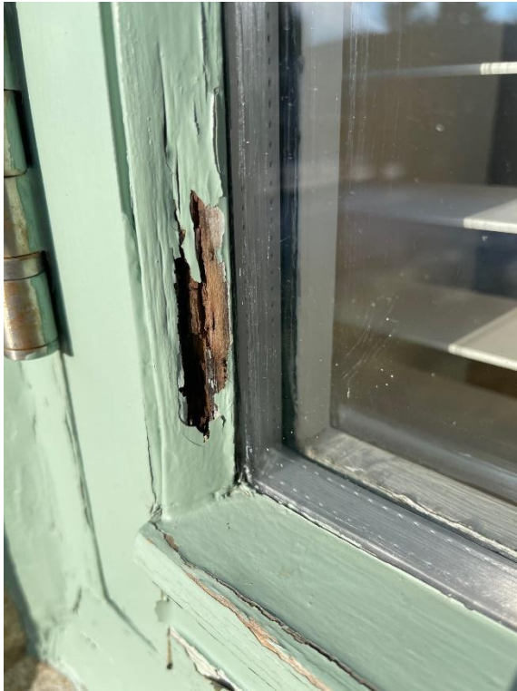
Existing rotting window frames at the application property
