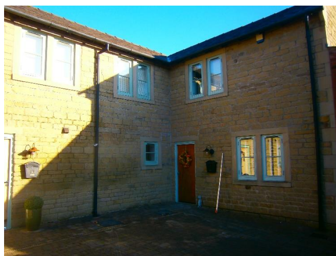
Northern elevation of dwelling
