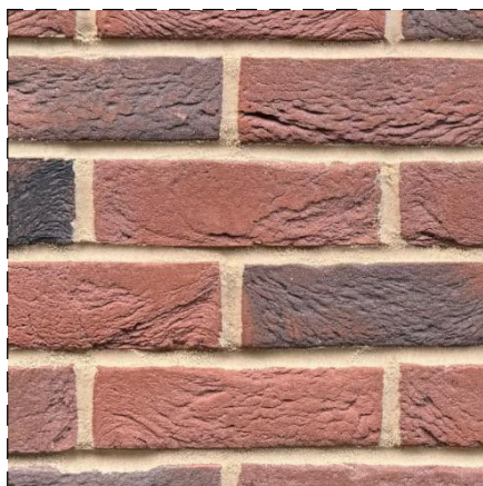
Lytham Multi Red Brickwork - External walls
