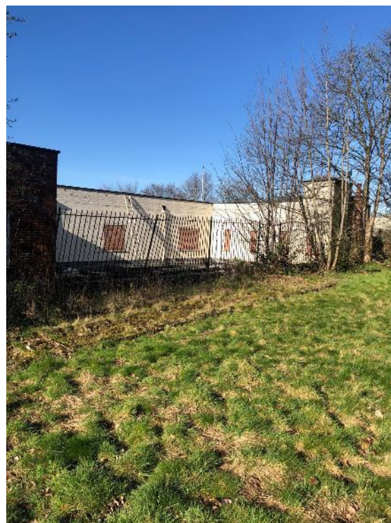
Photograph 4: Overview of the rear (north) elevation of the building observed from bowling green. No gaps recorded.
