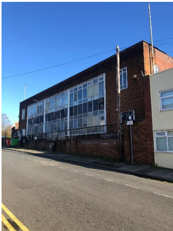
Photograph 1: Overview of the front (south) elevation of building. No gaps observed.
