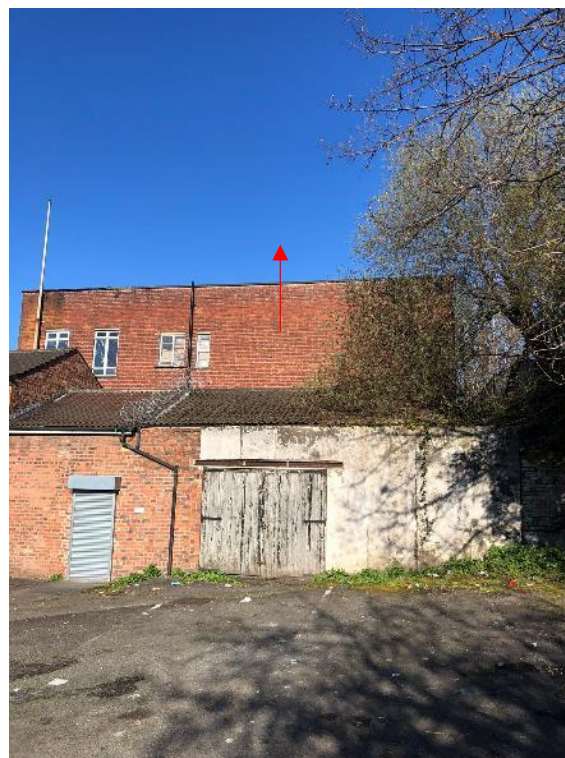
Photograph 3: Overview of the eastern aspect with no gaps recorded in brick work or around windows.
