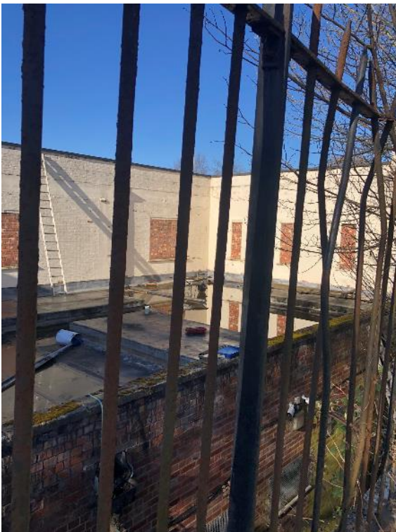
Photograph 6: Bitumen lined flat roof on single storey section. It is assumed that the two storey roof is of same construction.
