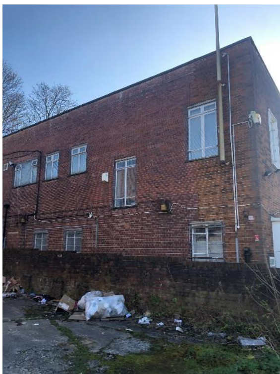
Photograph 2: Overview of the west elevation. Brick wall in good condition with no gaps recorded.
