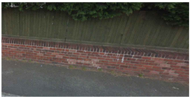
ADJACENT BOUNDARY WALL.
