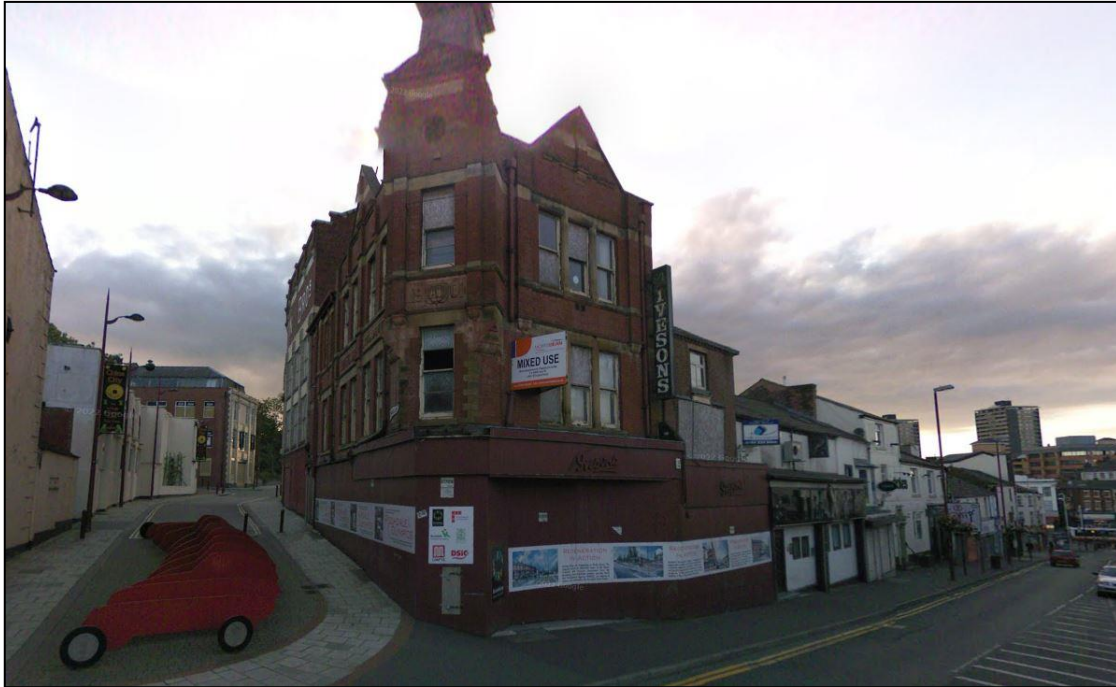
Figure 9: Trafalgar Buildings at the corner of Drake Street and Nelson Street c. 2008 (Google Street View)
