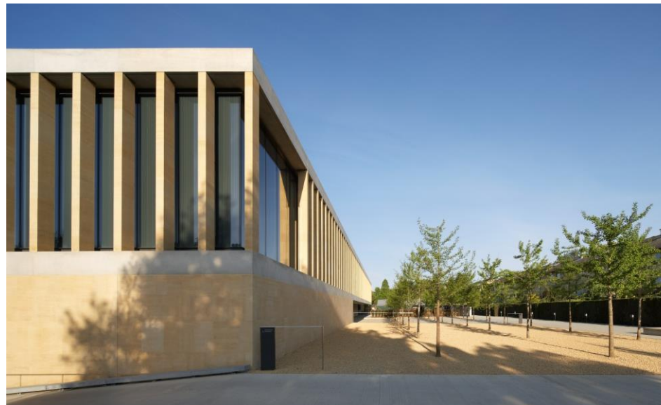
Johnsons Wellfield saw cut Pennine sandstone
