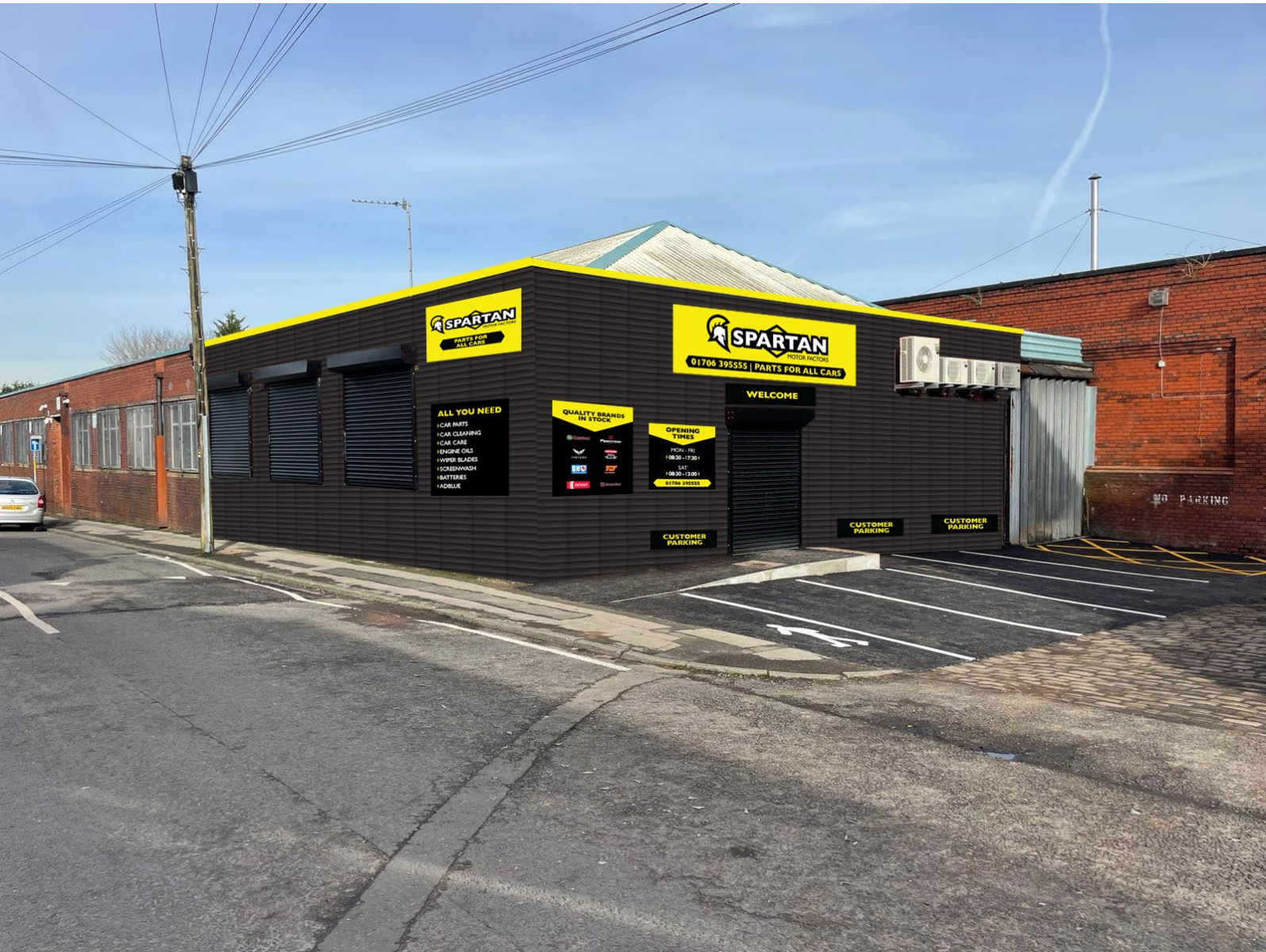
MOCK UP OF UNIT WITH SIGNAGE IN PLACE
