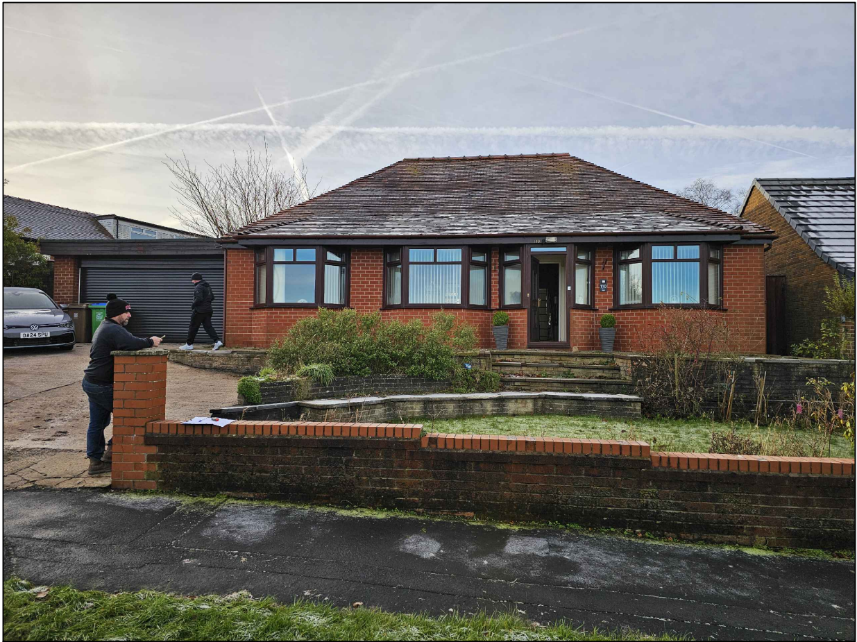
Site Photo-Existing Front Elevation
