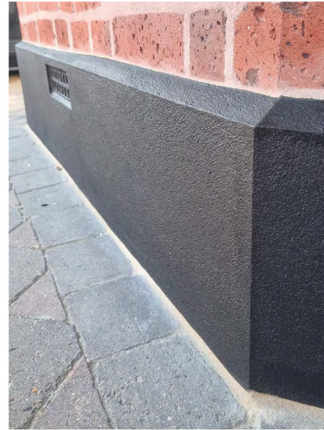
4 Rendered Plinth Detail Rough cast rendered finish. Colour: Black. Nominal height of 300mm (subject to local external levels).
