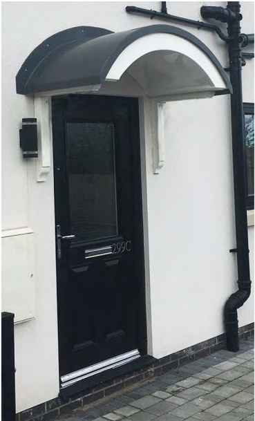
6 Entrance Door Canopies Colours: RAL 5014, 6033, 6018 (to match corresponding door colour) Weathered finish to top with flashing at junction with Brickwork above.
