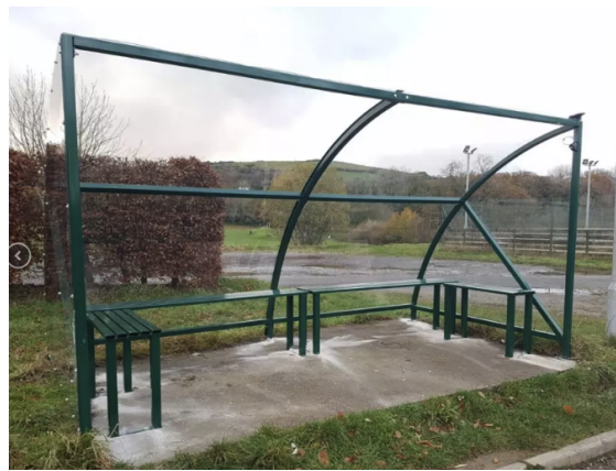
8.2 - Same profile shelter to be used for the smokers area
