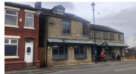
- Photo - indicating part front elevation & ridge line
