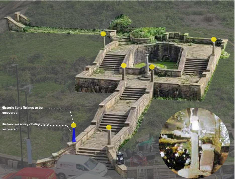
Image showing locations for missing obelisk lighting reinstatement
