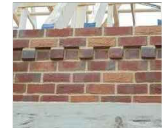
Eaves brick corbel detail -Butterley carbon black smooth
