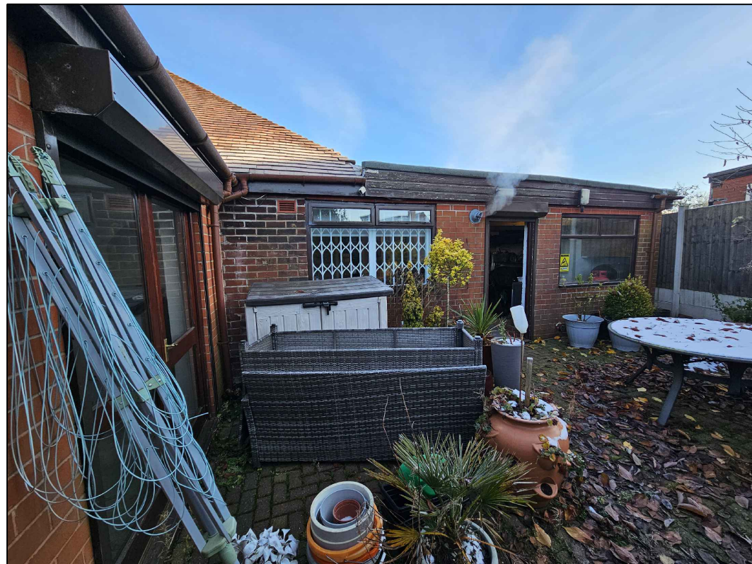
Site Photo-Part Existing Rear Elevation (View A)
