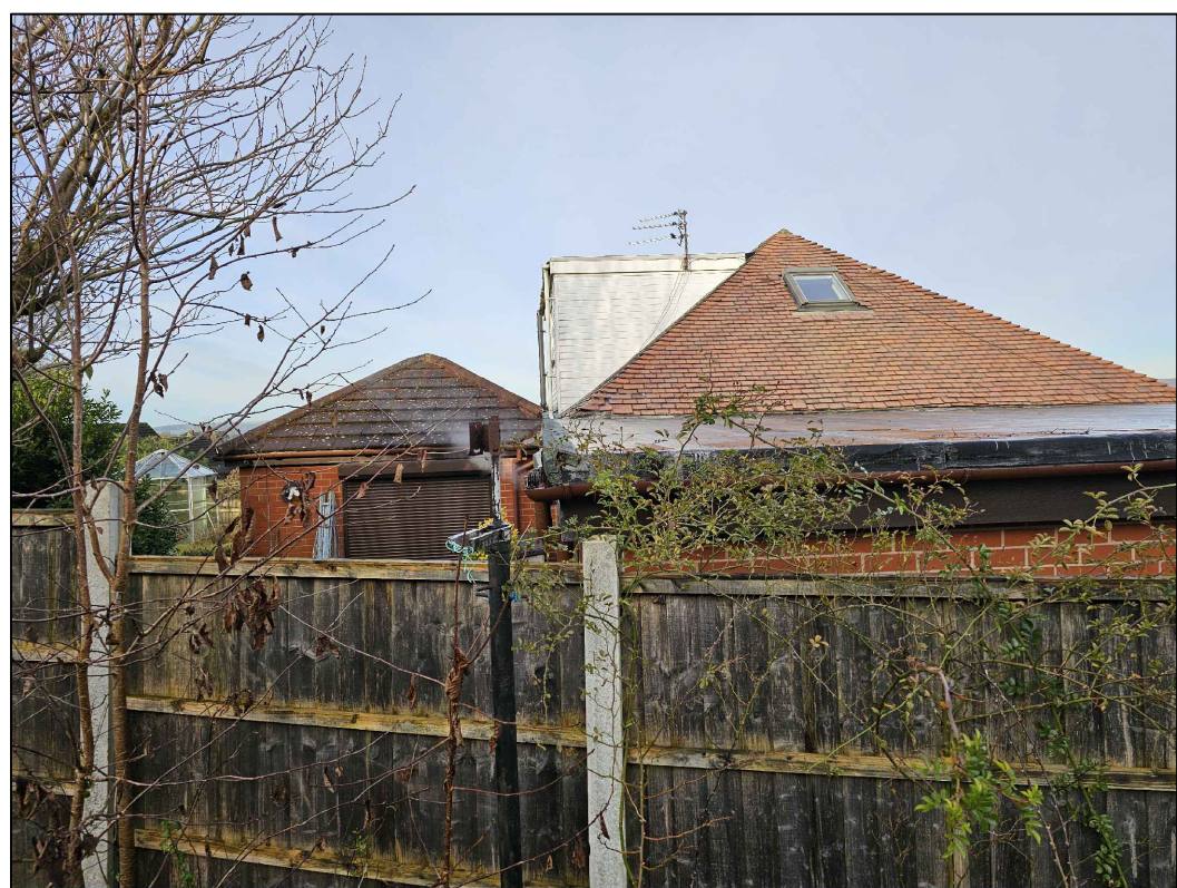
Site Photo-Part Existing South East Elevation
