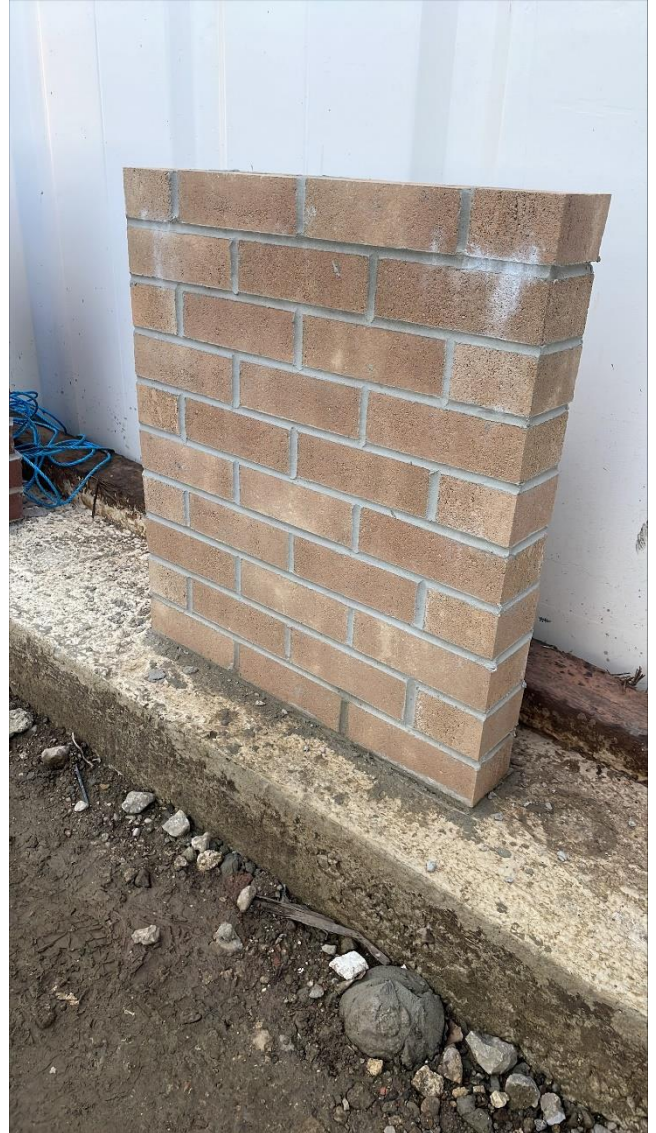
Brick Panel constructed on site.
