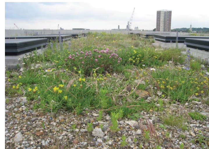
Extensive brown roof - aggregate with occasional plug planting
