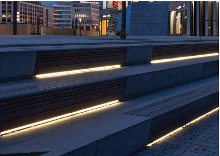
Under bench lighting
