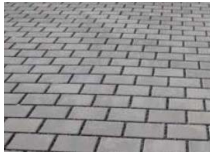
Car parking area
