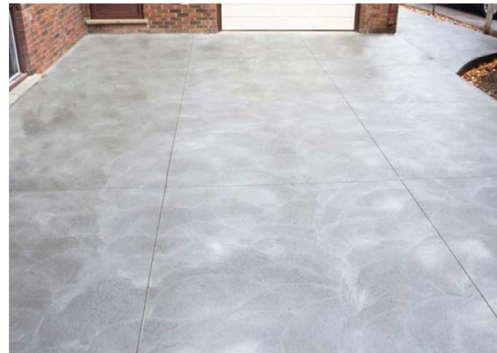
Poured concrete paving for the vehicular route
