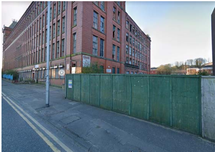
North-west entrance for the site
