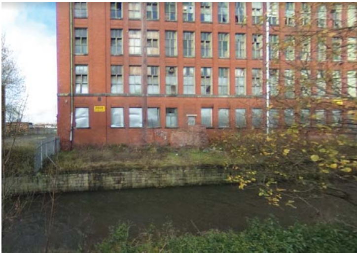
South-west corner of the site and the Wince Brook
