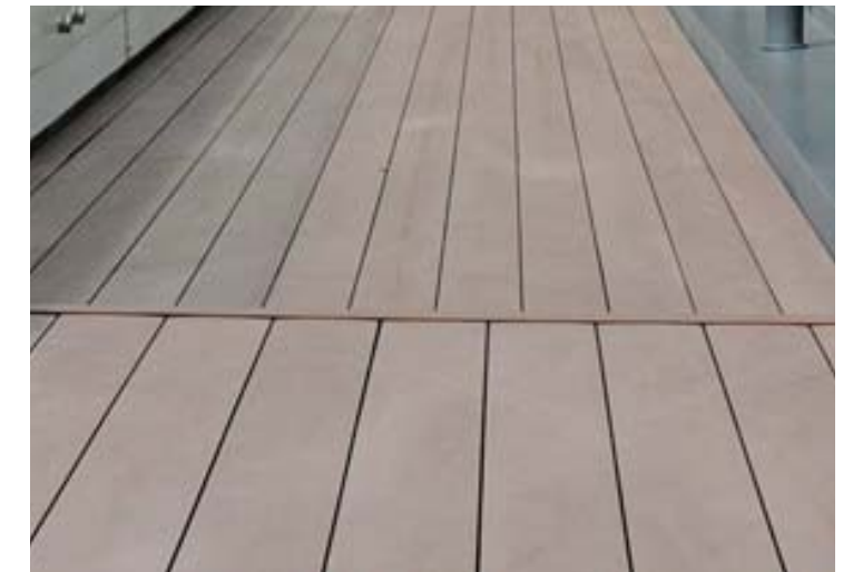
Decking to riverside and kitchen areas
