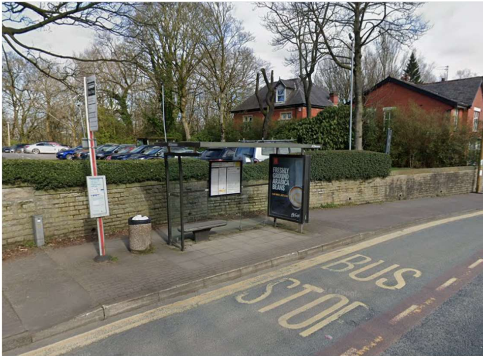
Northbound view of existing shelter
