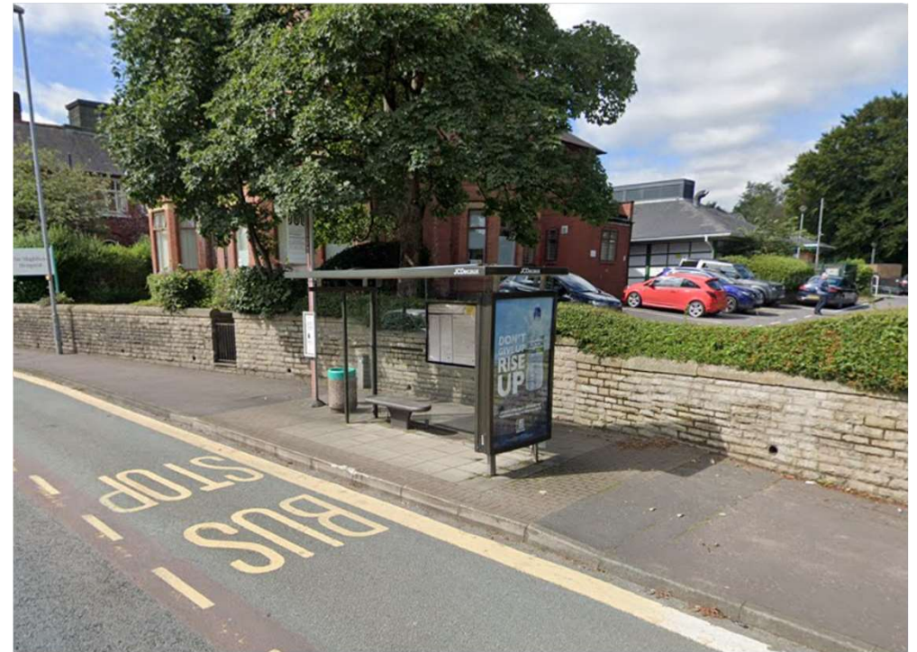
Southbound view of existing shelter
