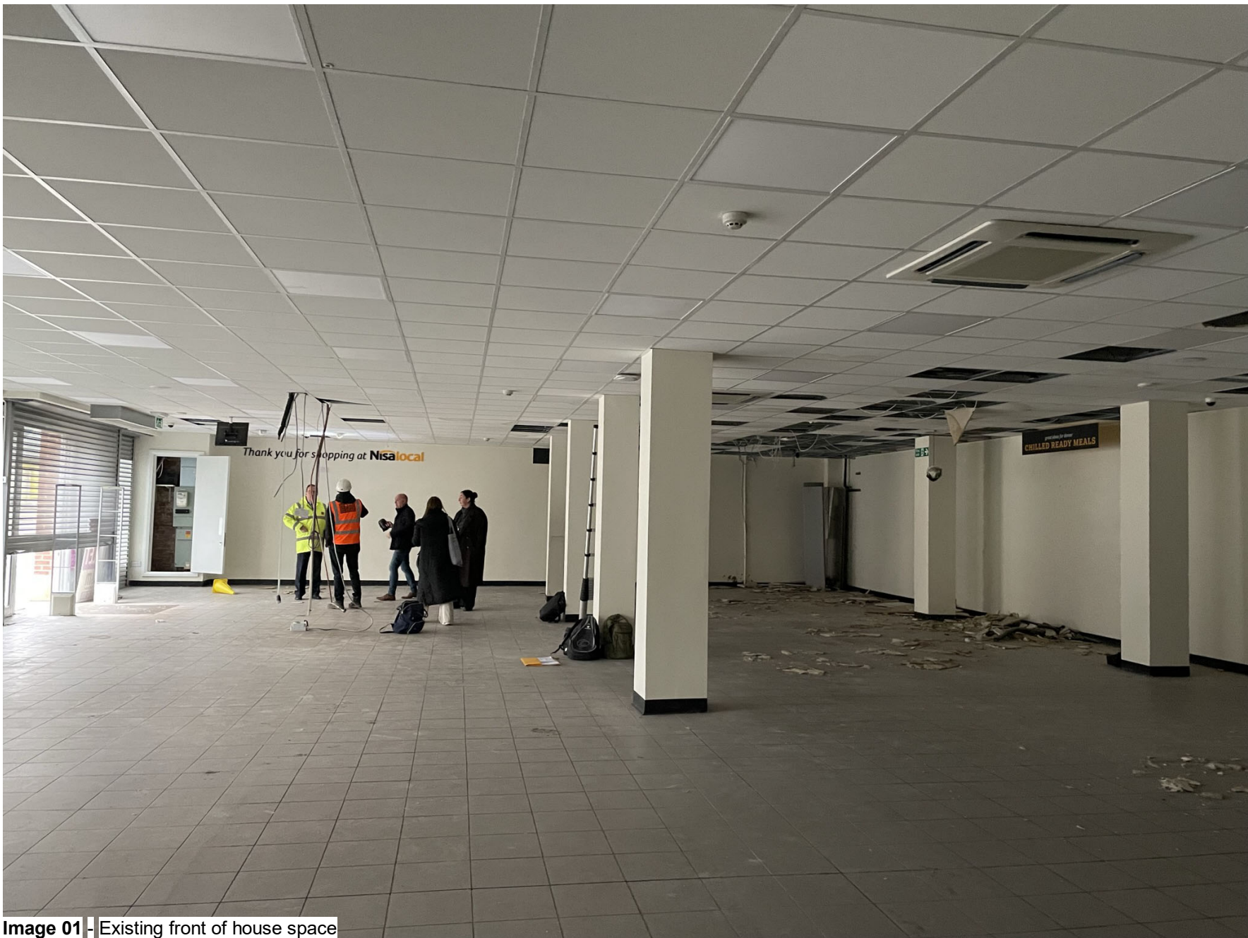
Image 01 | Existing front of house space
