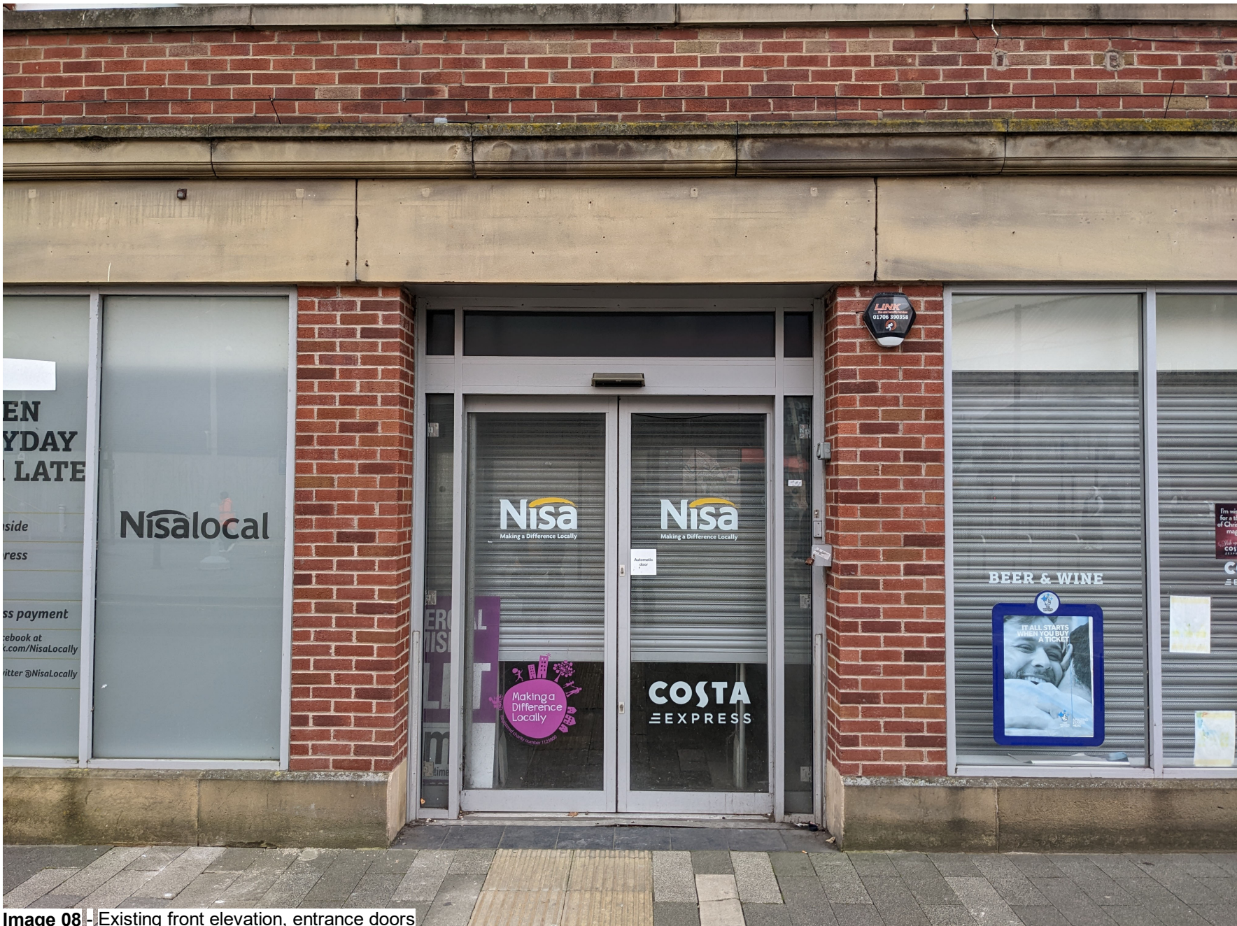
Image 08 | Existing front elevation, entrance doors
