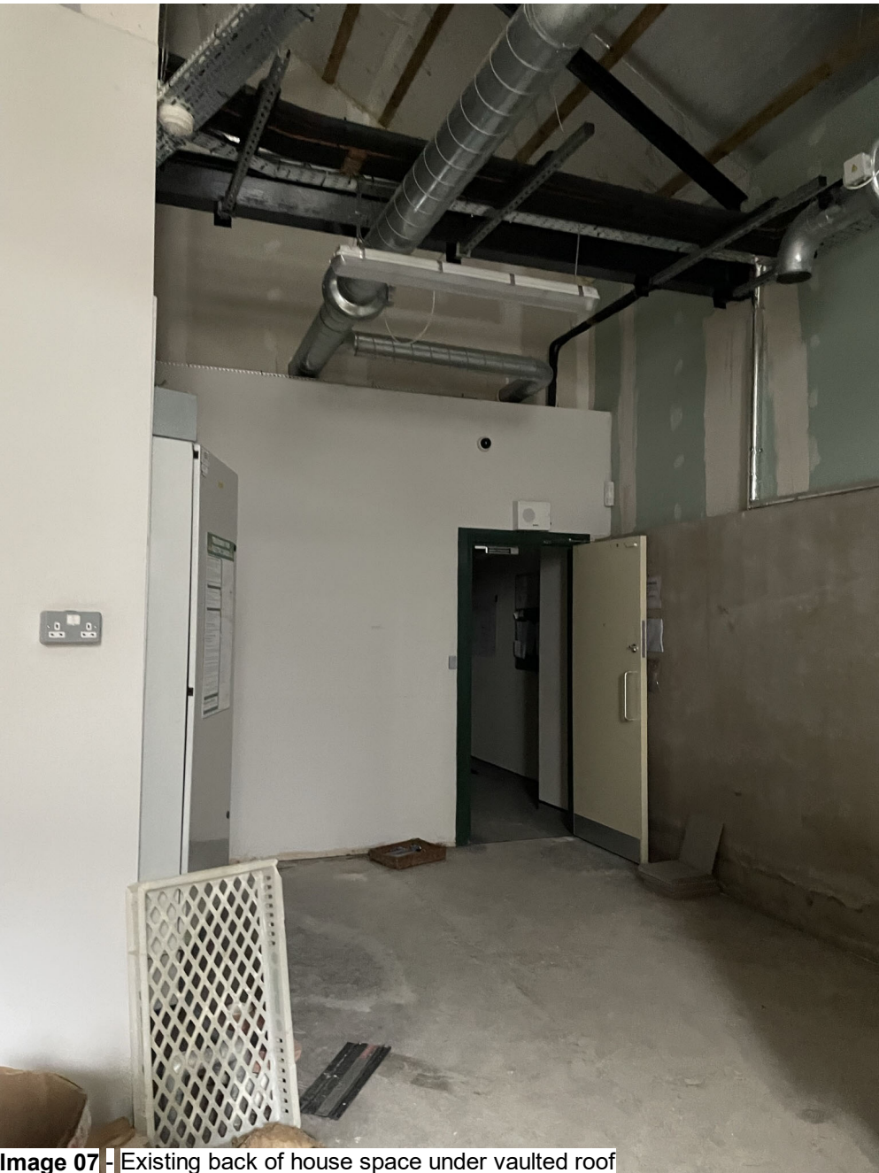
Image 07 | Existing back of house space under vaulted roof
