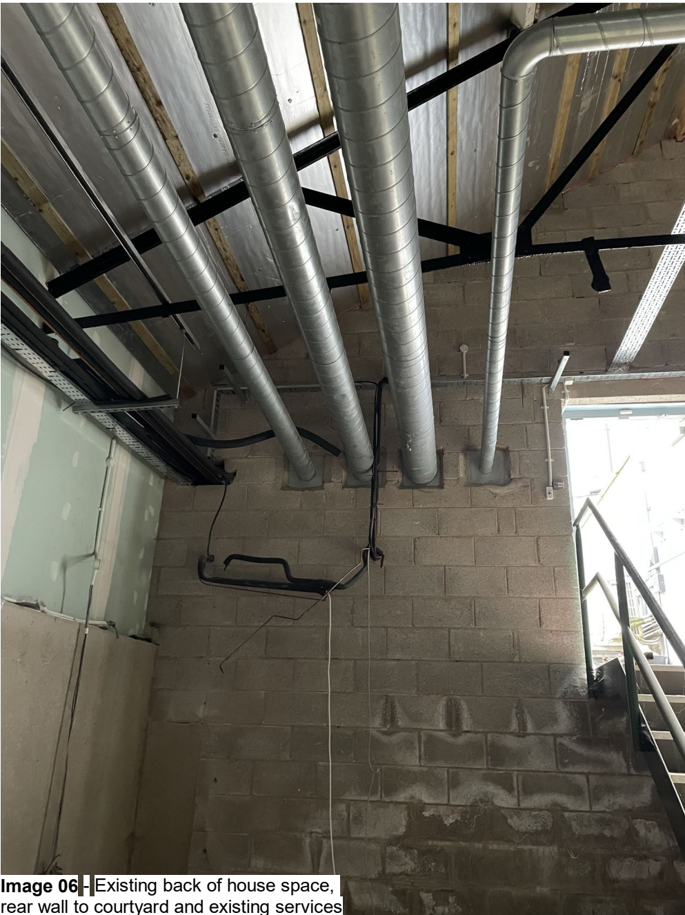
Image 06 | Existing back of house space, rear wall to courtyard and existing services
