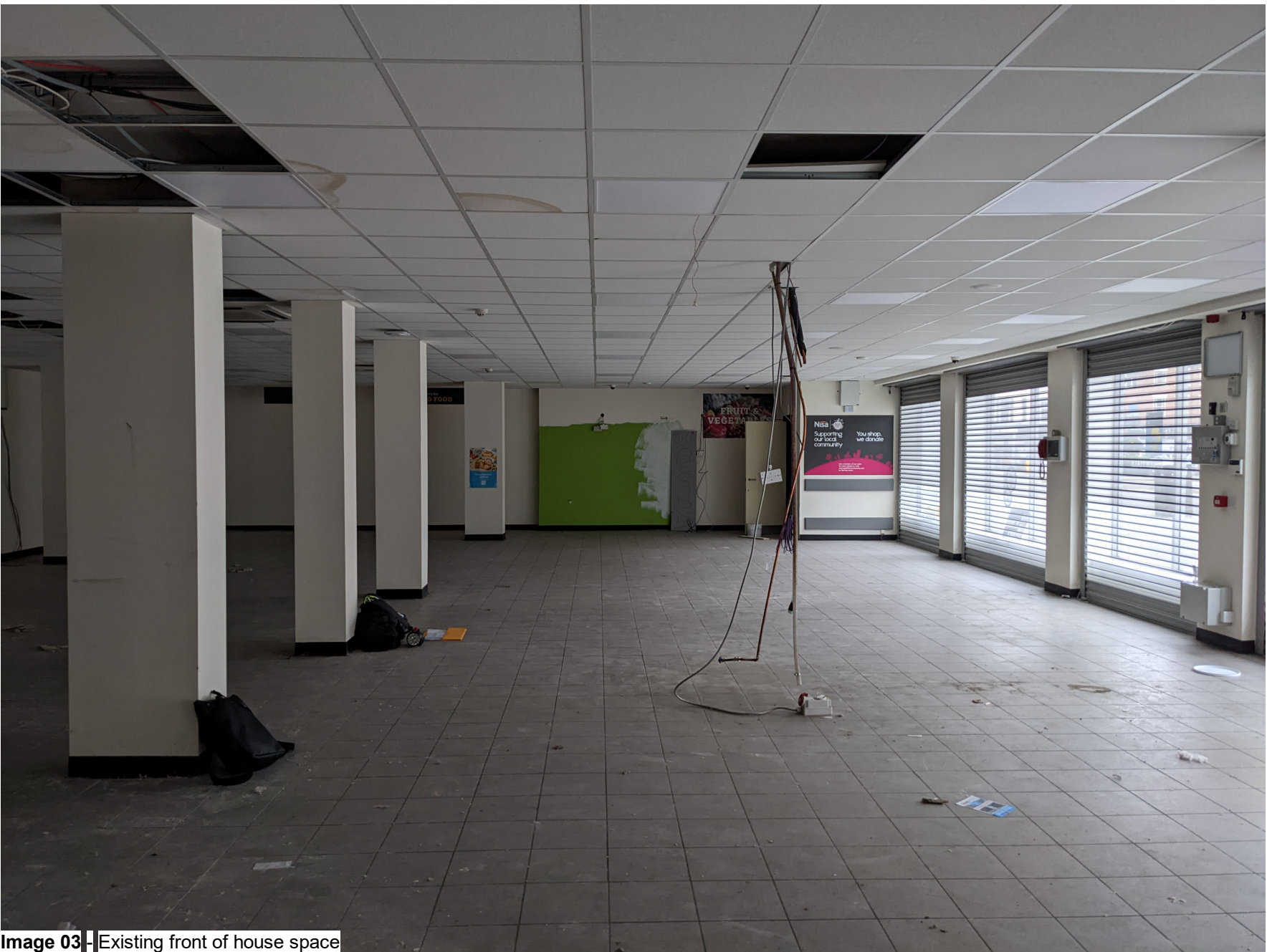
Image 03 | Existing front of house space
