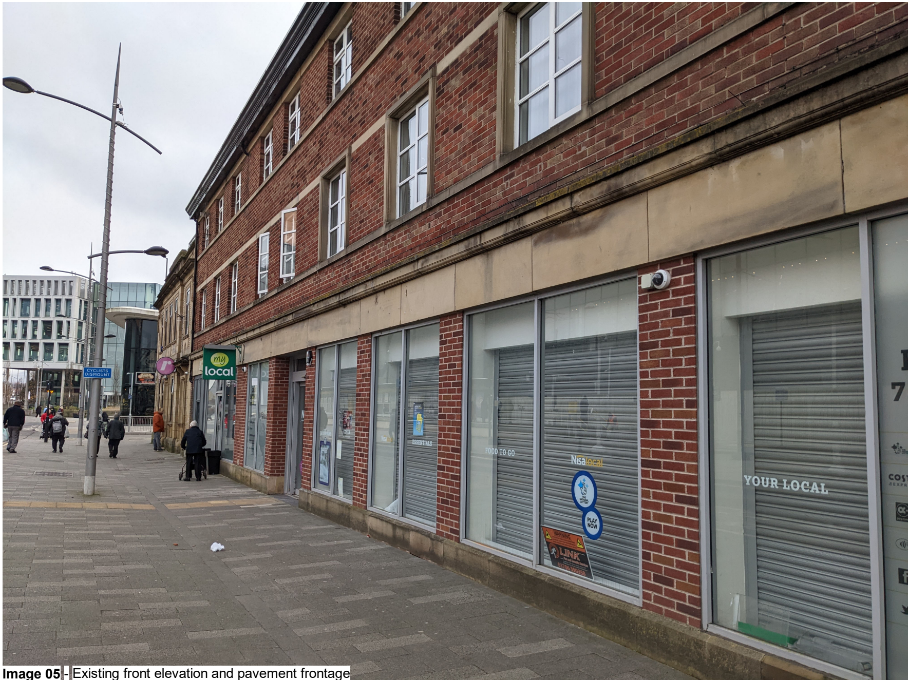
Image 05 | Existing front elevation and pavement frontage
