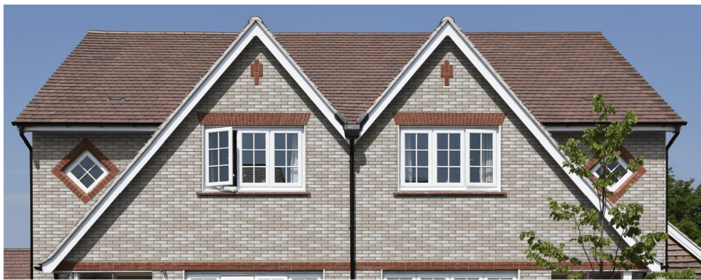
Ibstock Montpelier A5164A (Black Mortar) on stretcher bond
