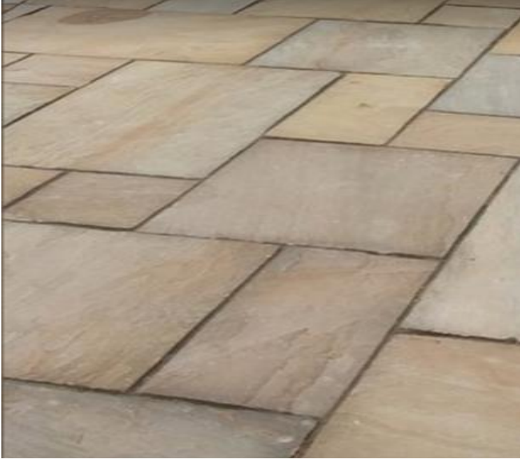
Buff Indian sandstone paving flags around building.
