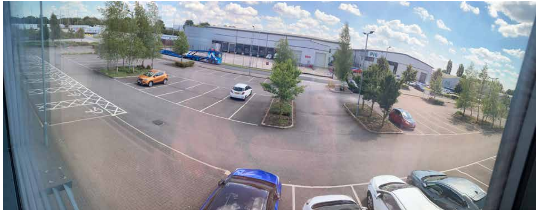
Existing carpark and entrance conditions.
