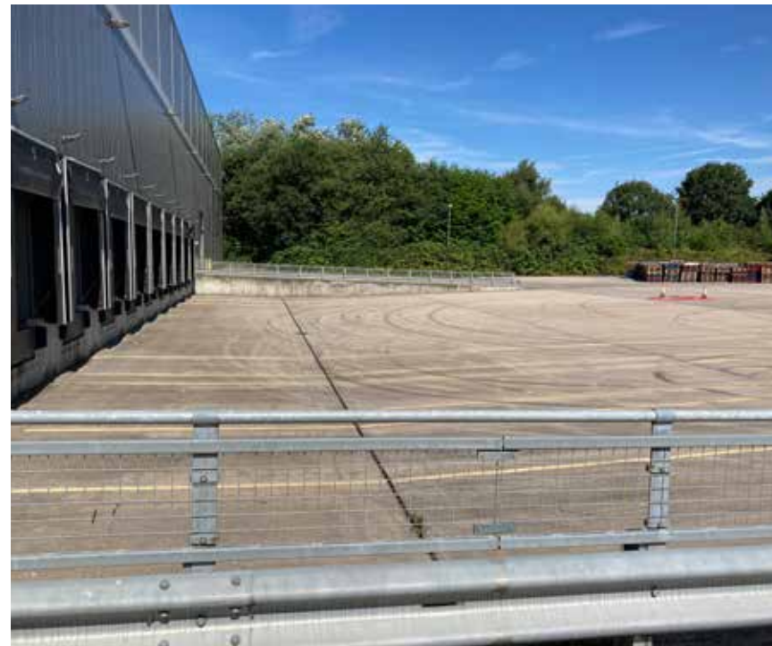
Image looking north of service yard.
