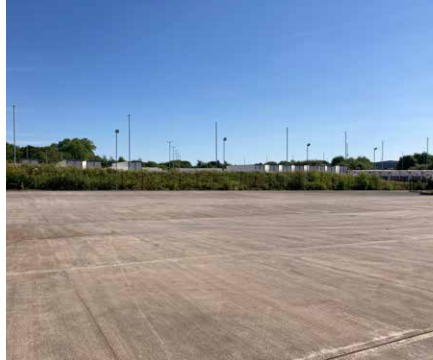
Existing service yard.
