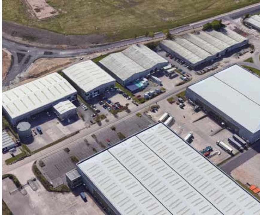
Aerial of adjacent buildings.
