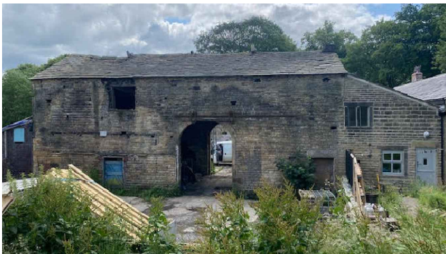
Existing Rear Elevation (photo)
