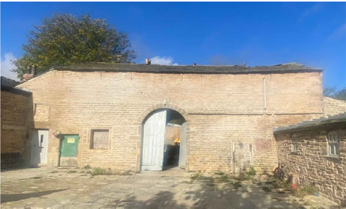
Existing Front Elevation (photo)
