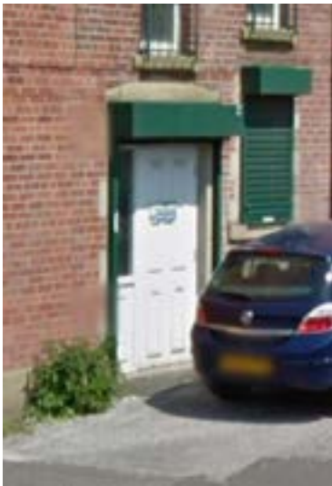
Existing side entrance.
