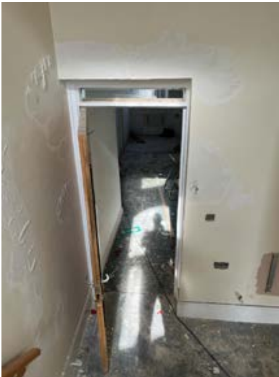
Picture of wall area for proposed entrance to bedroom 1.
