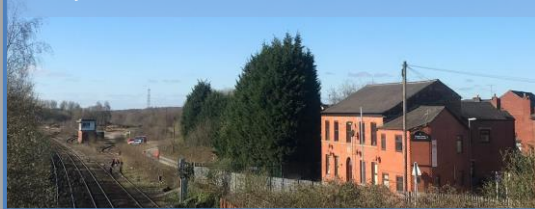
Looking south towards the site from the bridge over the railway at Manchester Road
