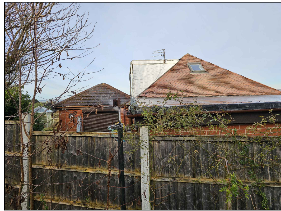
Site Photo-Part Existing South East Elevation
