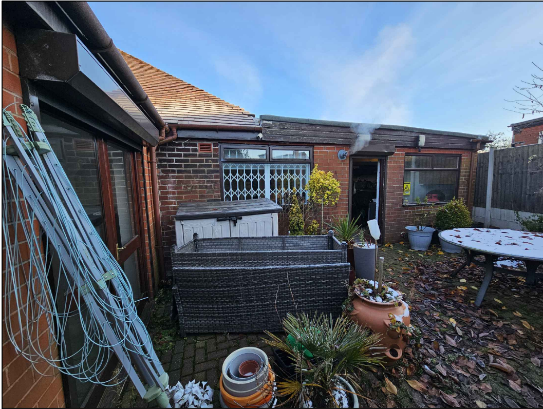
Site Photo-Part Existing Rear Elevation (View A)
