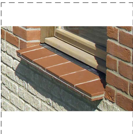
Terracotta Crease Tiles - External cills (Rear Elevation)
