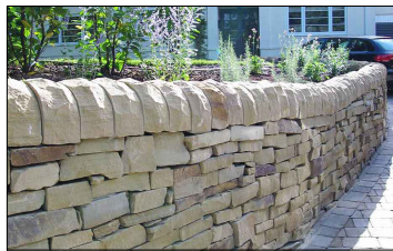
12. dry stone wall (re-built)
