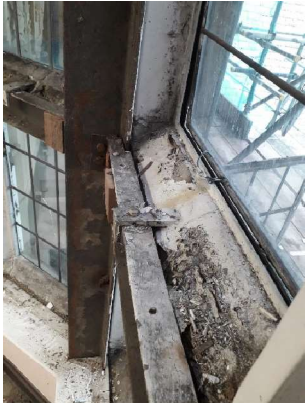
Upper oriel support frame exposed for inspection
