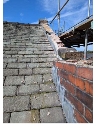
Copings removed for re-bedding and lining
