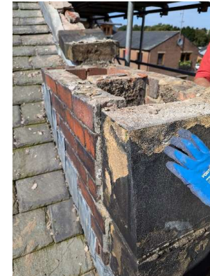
Chimney dismantled to sound brickwork and flues inspected
