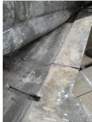
Gutter stonework uncovered for inspection
