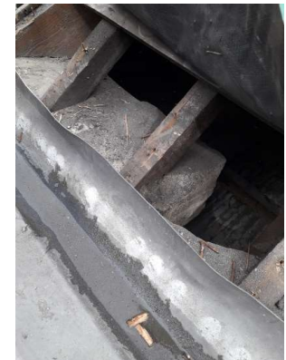
Oriel roof structure supported and exposed
