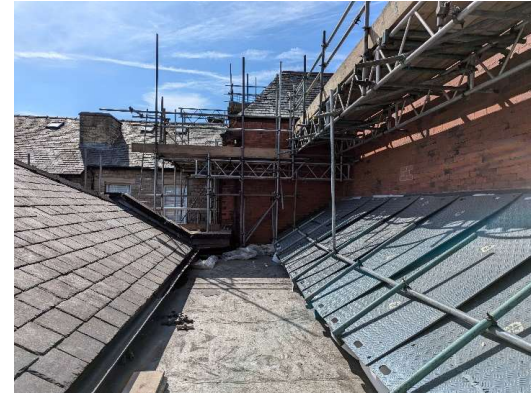
Skylight protected and flat roof inspected/works agreed
