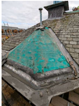
Oriel Roof stripped to reveal structure
