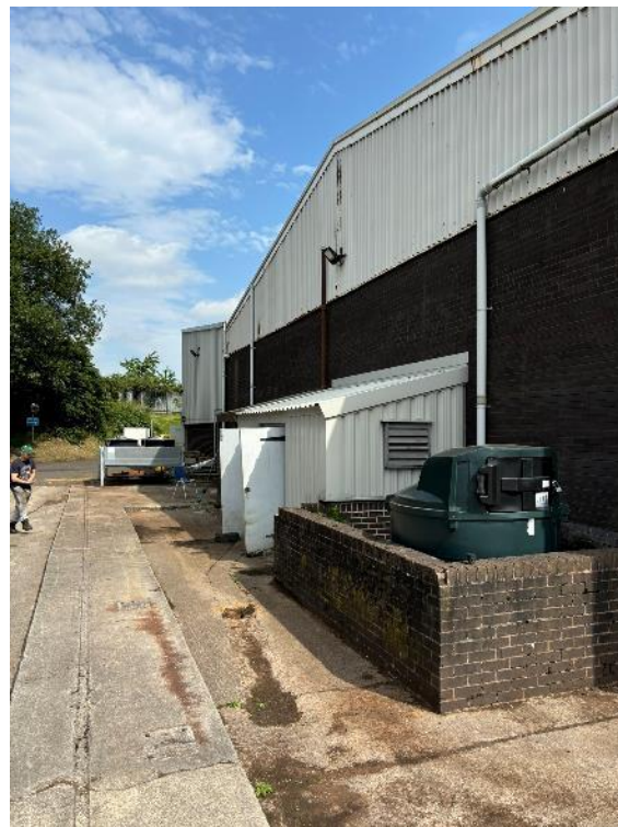
Photograph 3: View along the western elevation. Security lighting along entire elevation. Negligible.
