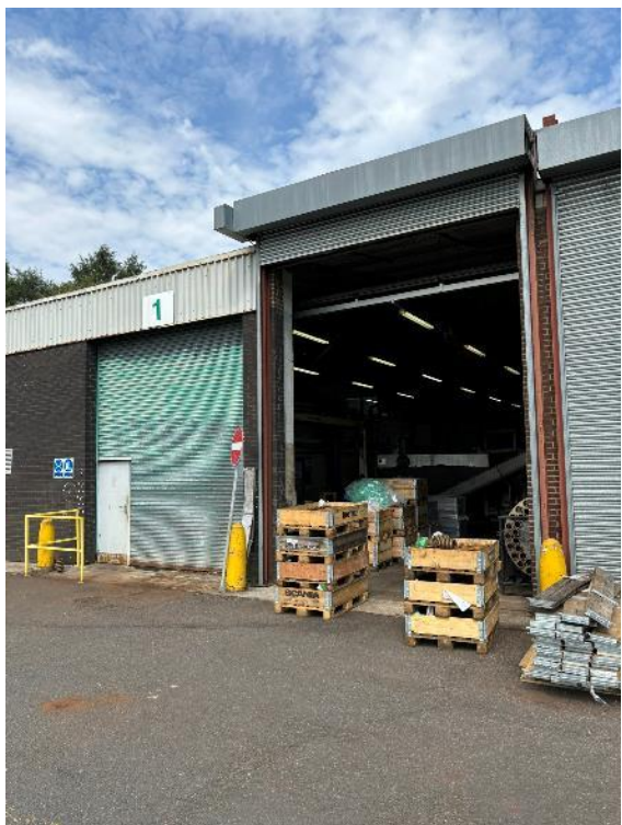
Photograph 2: Overview of the south (front) elevation where the extension is proposed. Negligible BRP.
