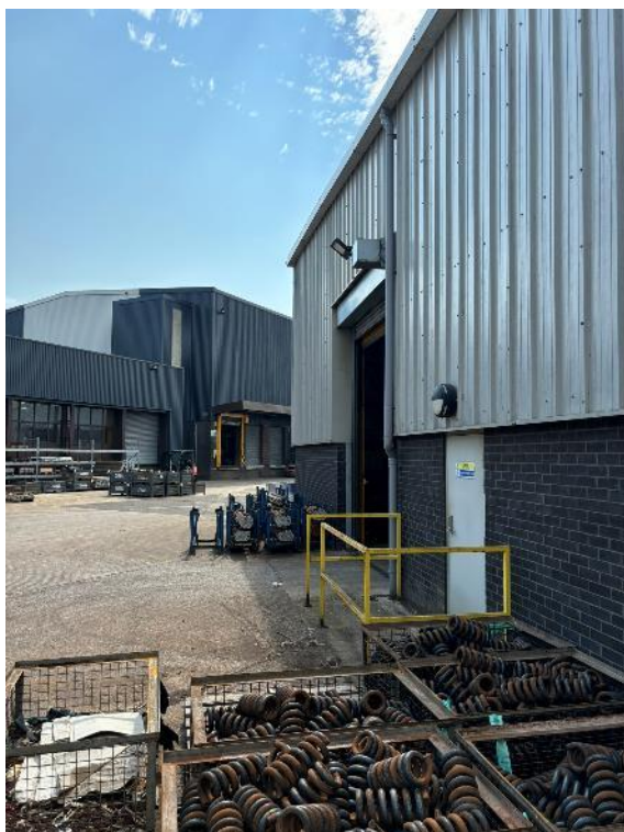
Photograph 6: Eastern elevation of building unaffected by proposals. Negligible potential.
