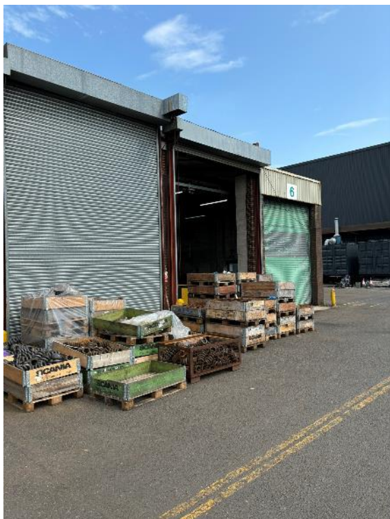
Photograph 1: Overview of the south (front) elevation where the extension is proposed. Negligible BRP.
