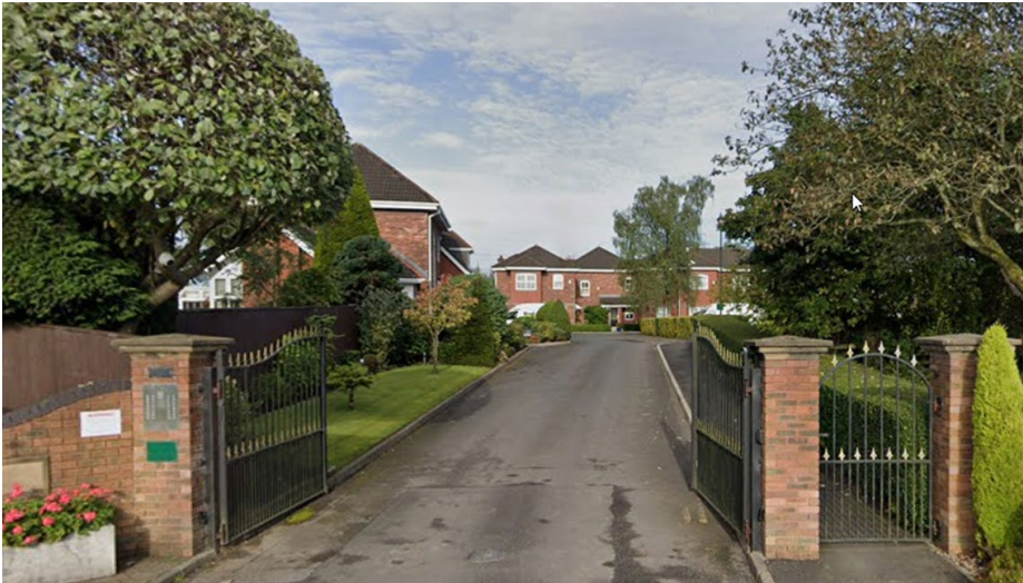
A View of the entrance to Bamford Mews and the site.
