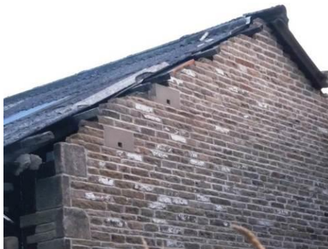
Example of Forticrete boxes in situ
