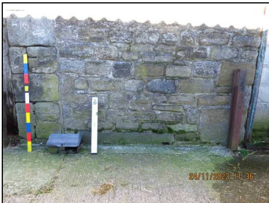
027 Ground floor, chainage 5 – 10 metres
