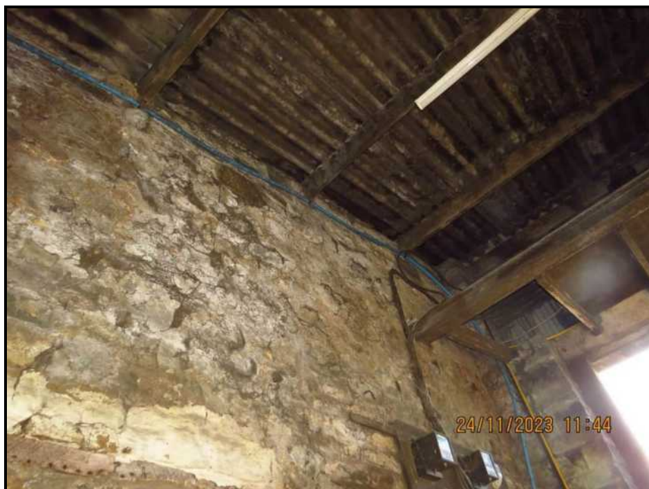
051 Eastern gable, front corner
