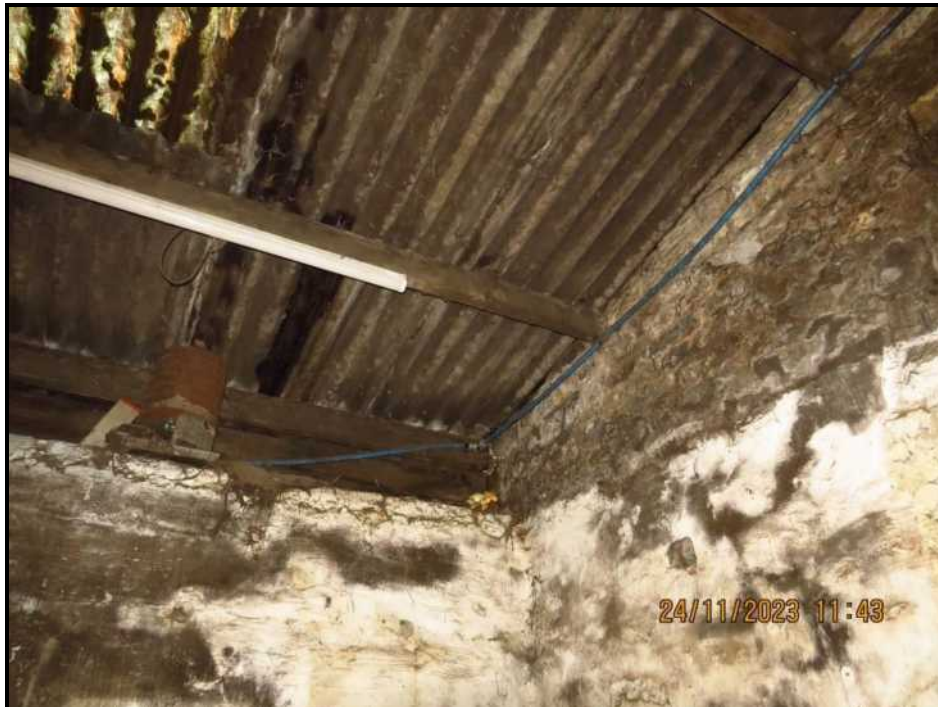
043 Roof, Northern corner
