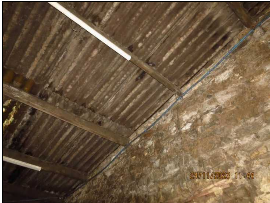
050 Eastern gable, roof support
