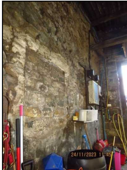
Photograph 053 Former window, internal corner South/East
