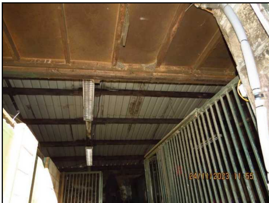
088 Roof, front elevation
