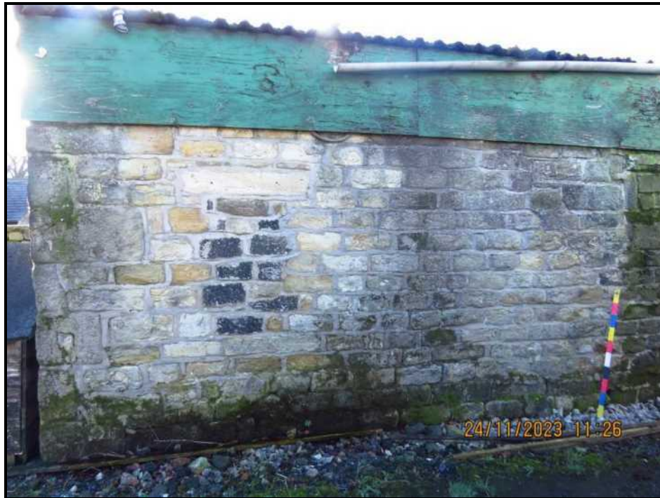
012 Rear wall, chainage 0 – 4 metres
