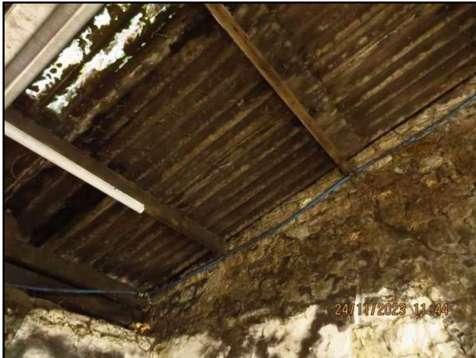
045 Purlin seating, Eastern gable
