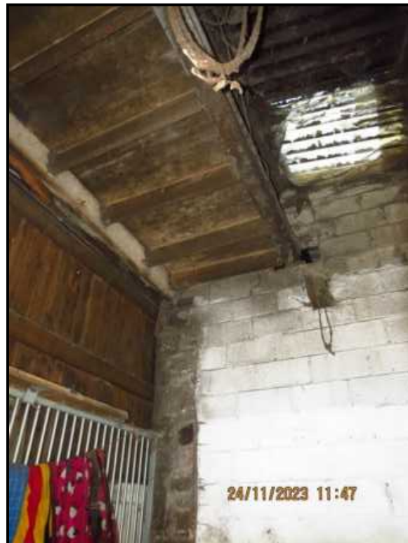
059 Front elevation, upper roof and cross wall
