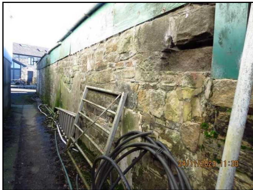
Photograph 020 Rear elevation looking South East
