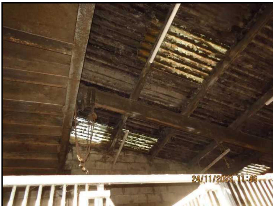
057 Internal cross wall to Stable No. 2
