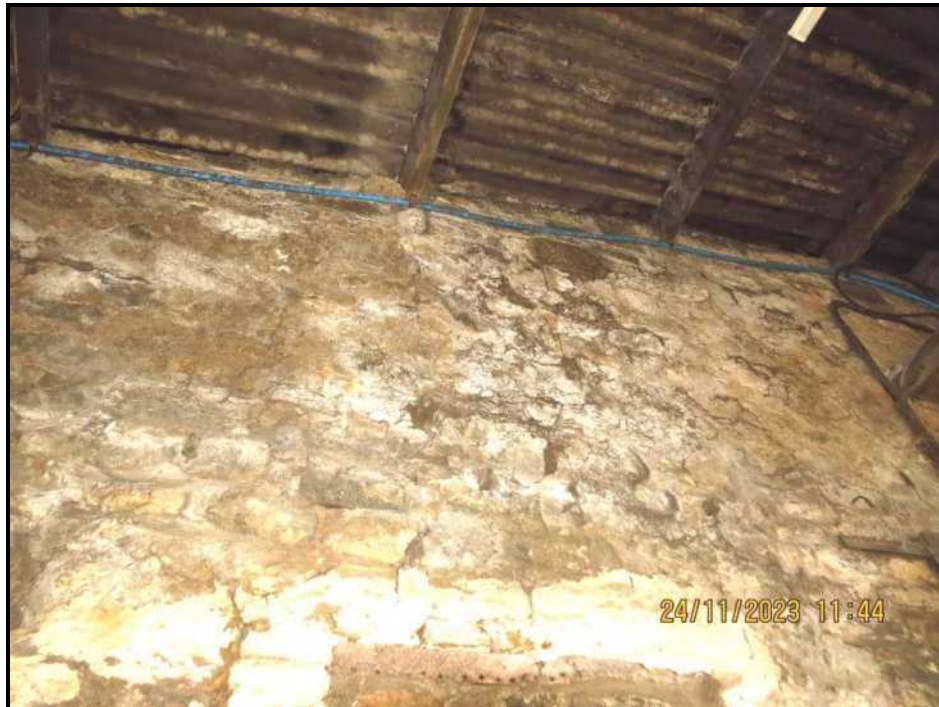
052 Upper wall, East
