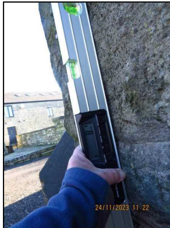
010 Good vertical alignment 8mm per metre
