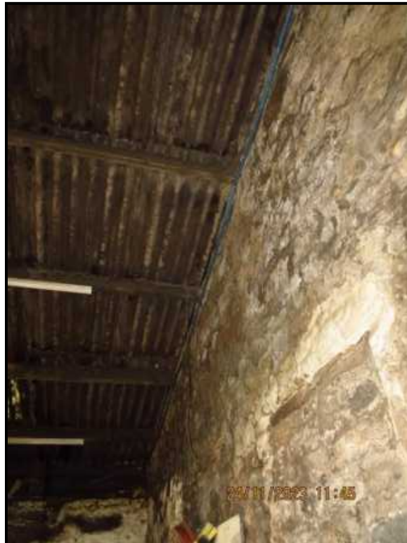
055 Gable elevation looking to rear
