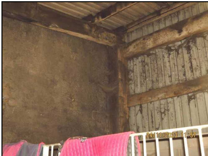
Photograph 093 Outside of West wall
