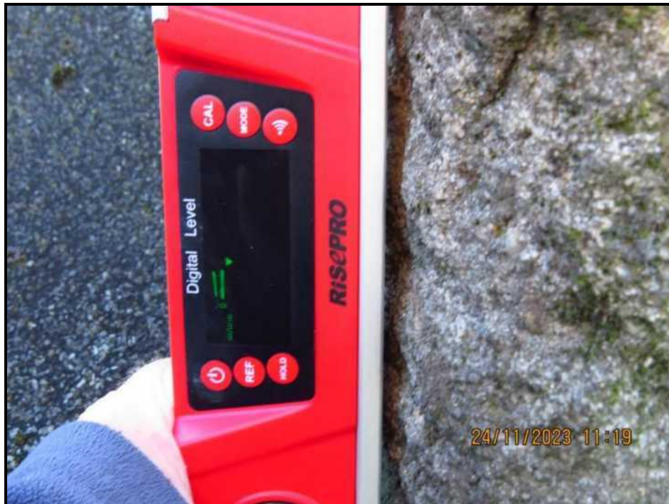
007 Satisfactory vertical alignment 5mm per metre
