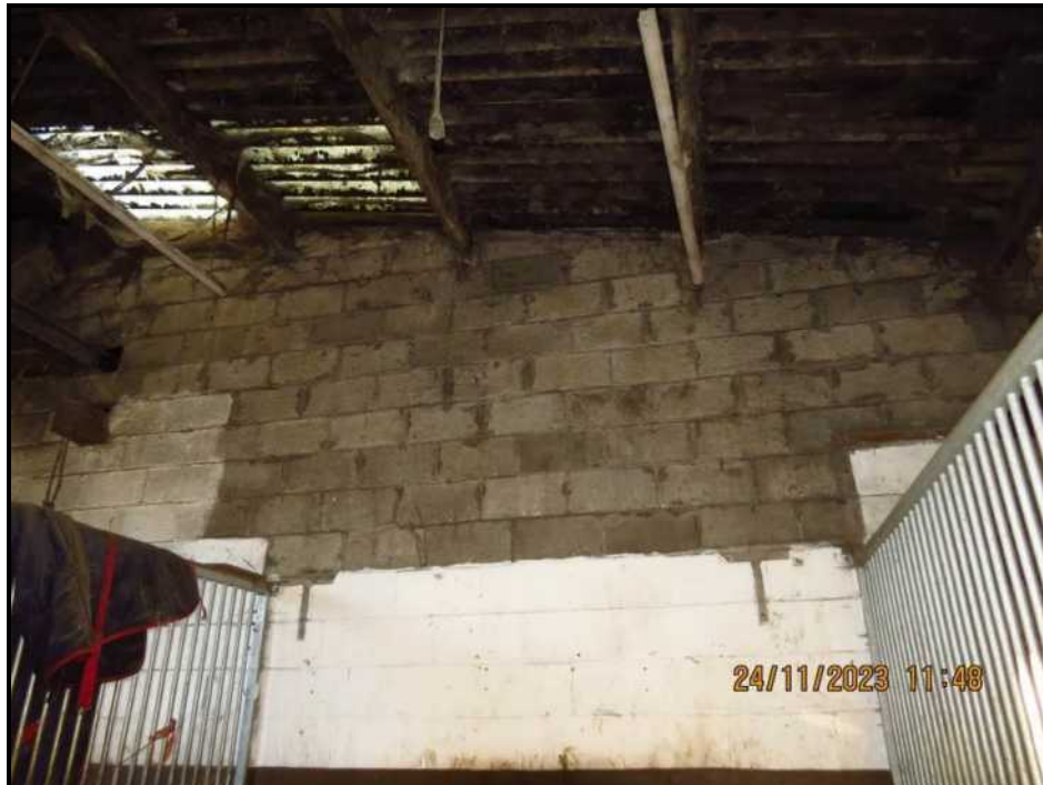
062 Internal party wall with Stable No. 2
