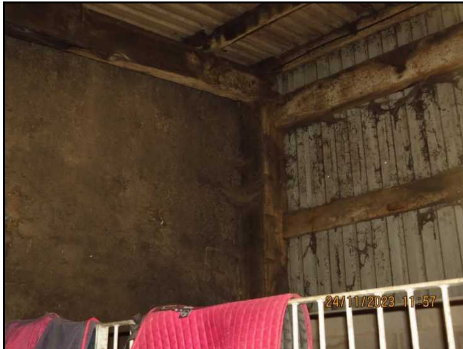
093 'Outside' of Western wall
