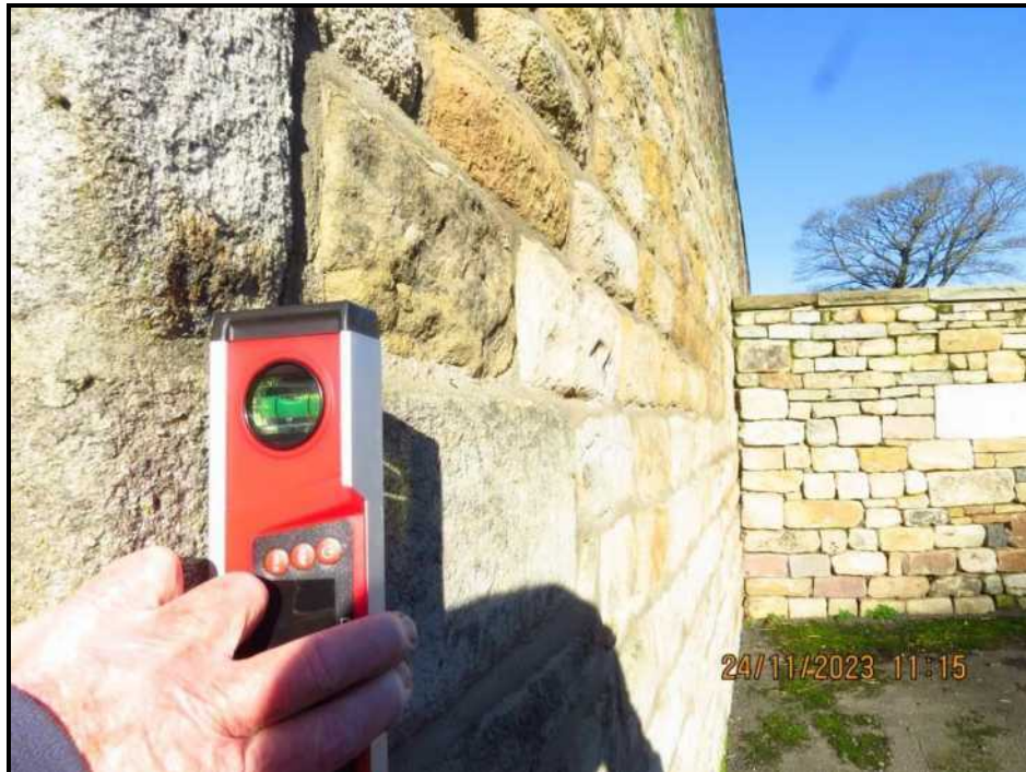
003 Satisfactory vertical alignment
