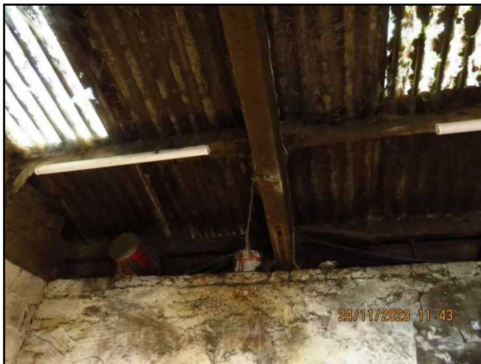
042 Rear wall rafter beam
