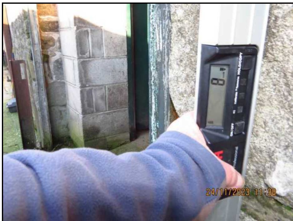
031 Good vertical alignment
