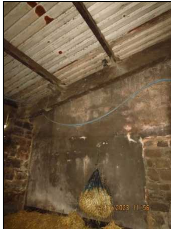
090 'Outside' of Western wall
