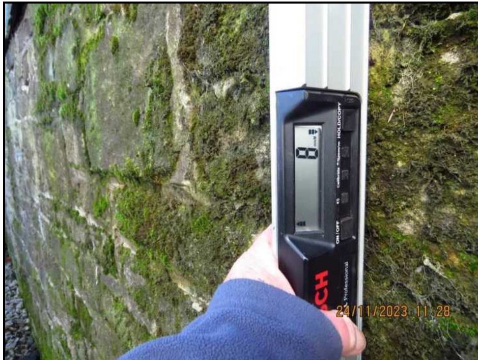
016 Satisfactory vertical alignment, chainage 12 metres
