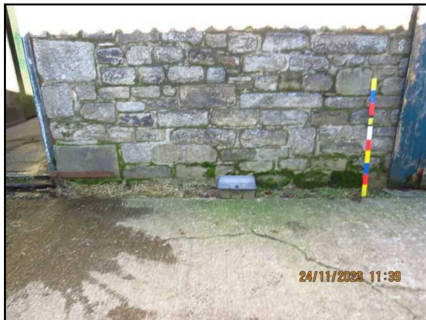
Photograph 032 Plinth wall, chainage 10 – 7 metres
