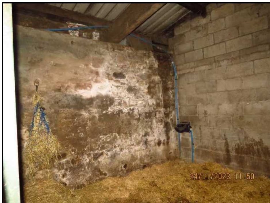
072 Rear wall and party wall, North East corner
