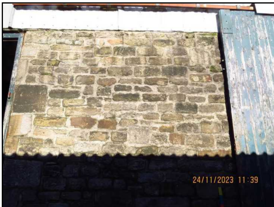
033 Upper wall, chainage 10 – 7 metres
