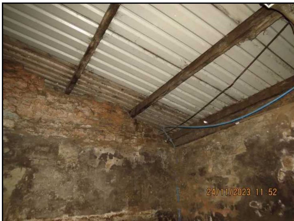
076 Western cross wall/rear wall
