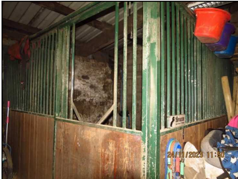
071 Stable No. 2 rear wall
