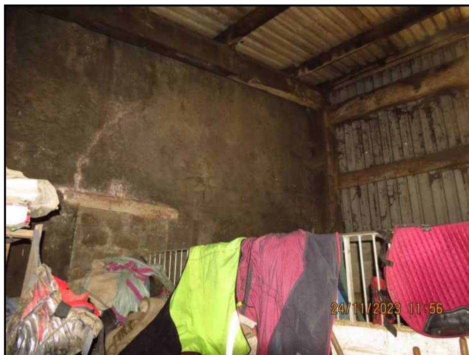
092 'Outside' of Western wall
