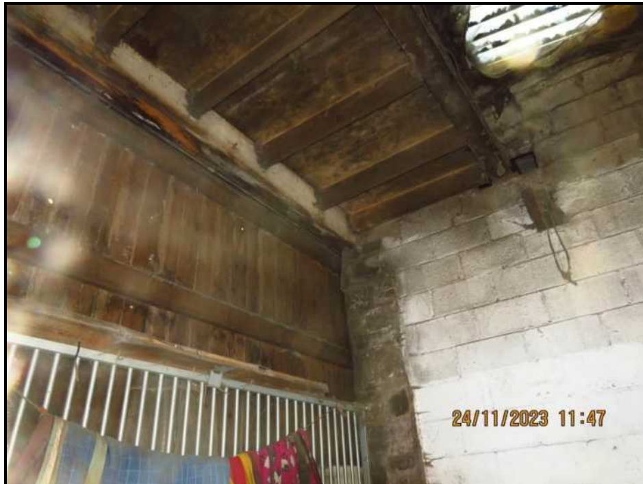
060 Front elevation, upper roof and cross wall
