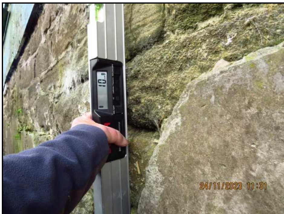
021 Satisfactory vertical alignment, \pm 5\text{mm} per metre
