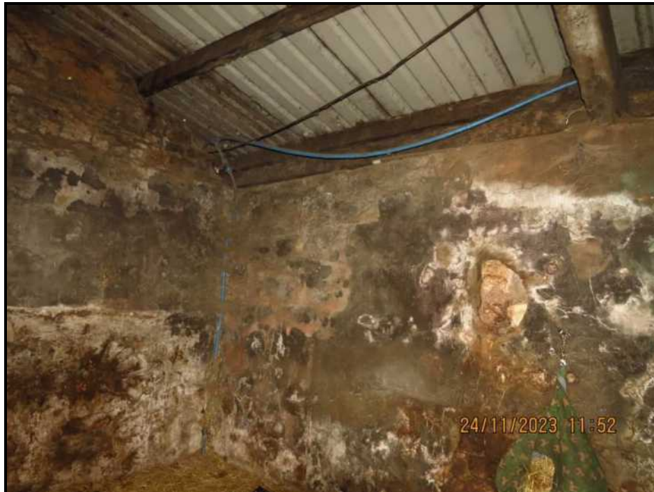
075 Rear wall Unit No. 2
