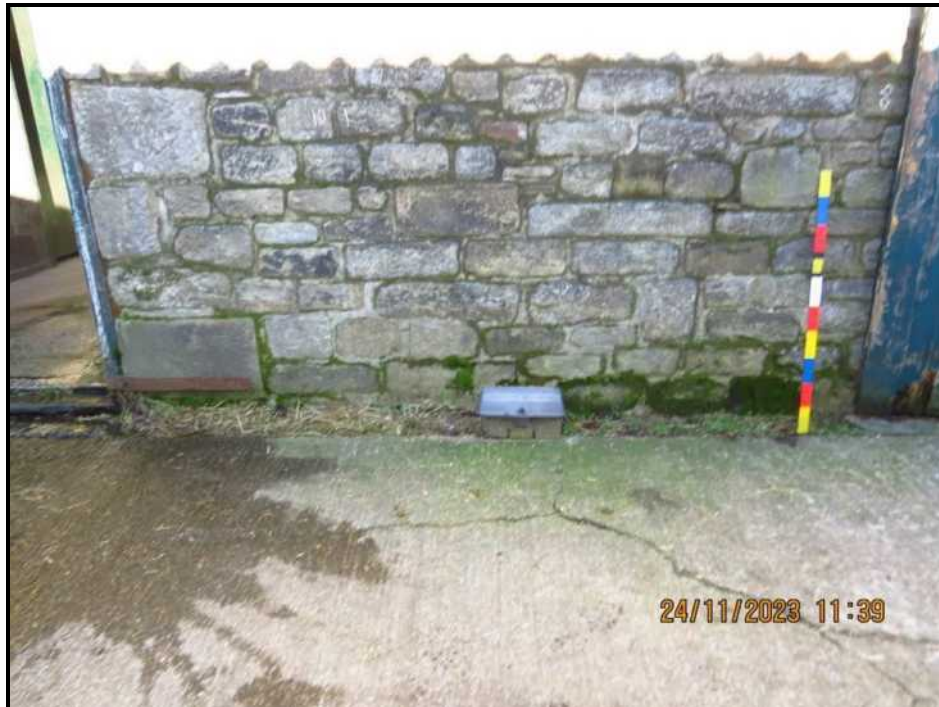
032 Plinth wall, chainage 10 – 7 metres
