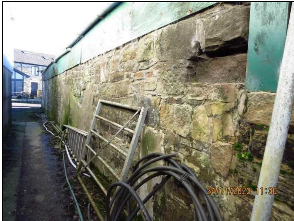
020 Rear elevation looking South East
