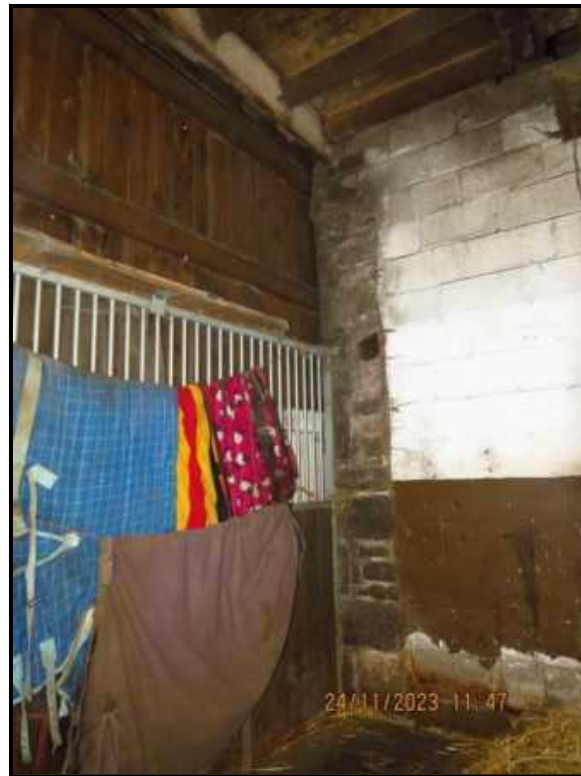
058 Front elevation and internal cross wall
