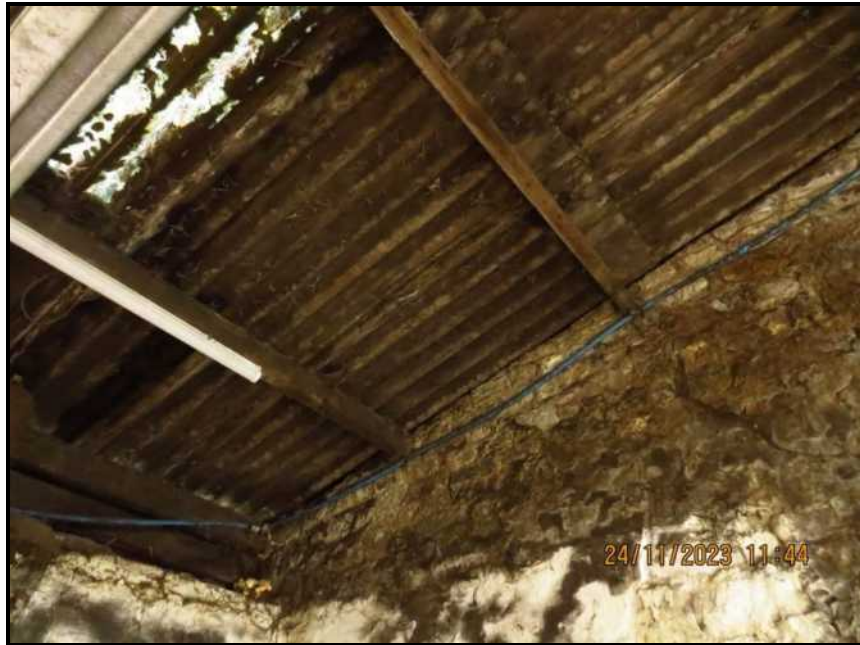
(Photograph 045 Purlin seating Eastern gable)
