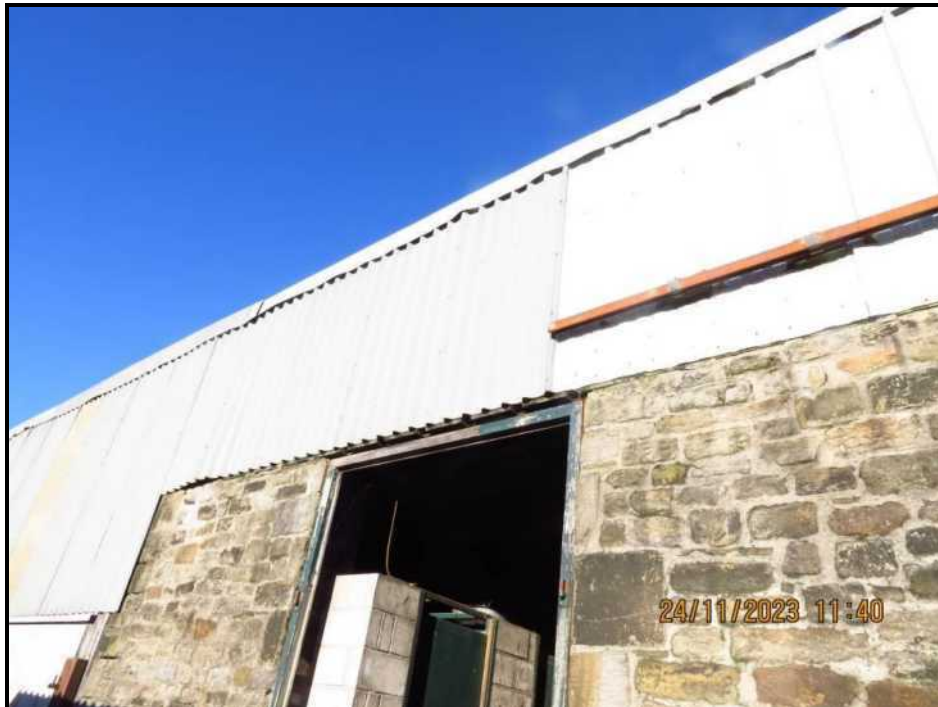
034 Upper wall, chainage 16 – 7 metres
