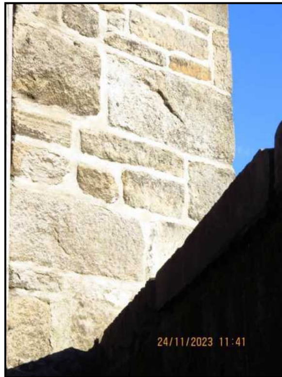
039 South Eastern corner, chainage 1.2 – 0 metres
