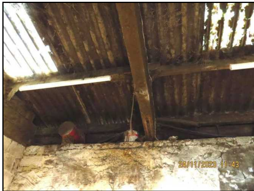
Photograph 042 Rear wall rafter beam
