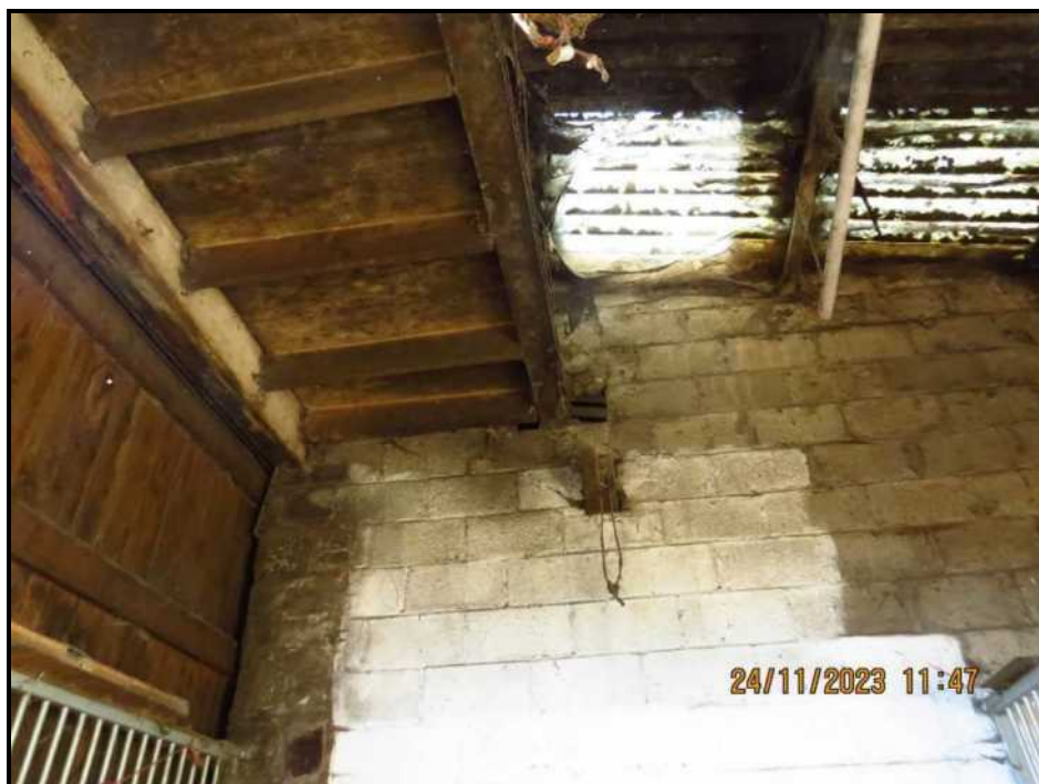
061 Internal party wall with Stable No. 2
