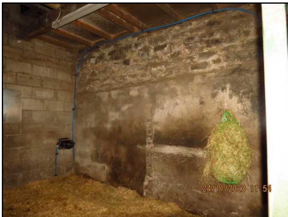
084 Party wall/front wall
