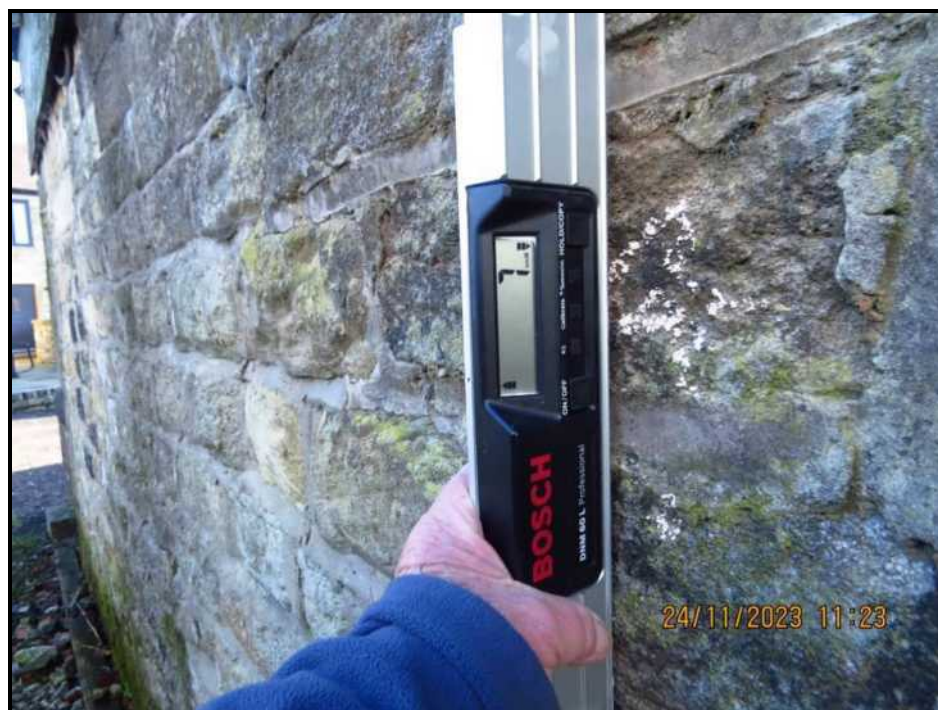
011 Chainage 4 metres, 7mm per metre
