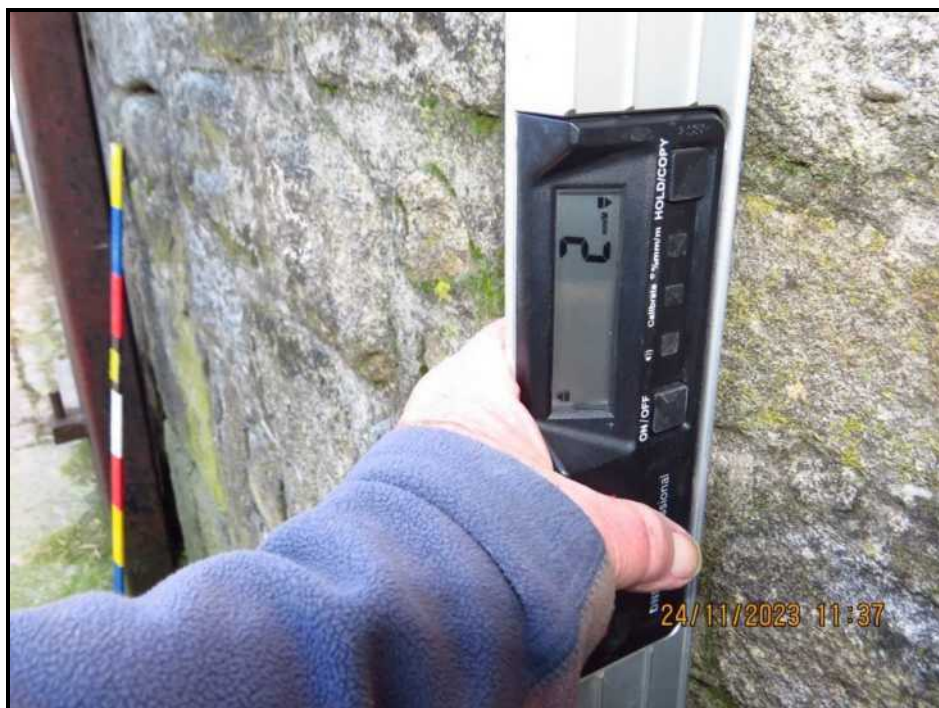
029 Good vertical alignment, 2mm per metre
