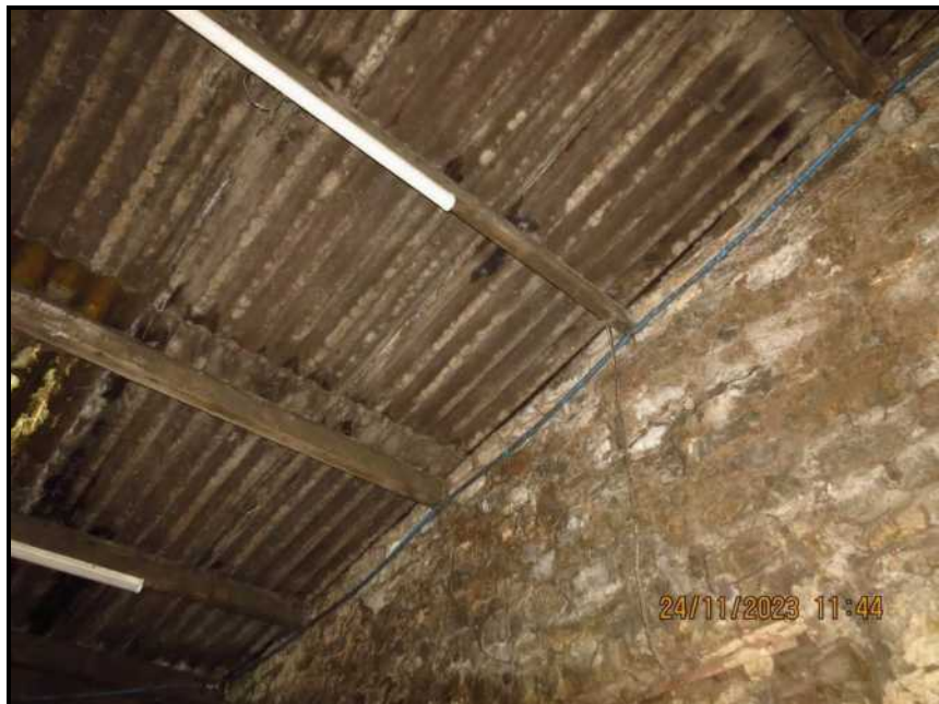
Photograph 050 Eastern gable roof support
