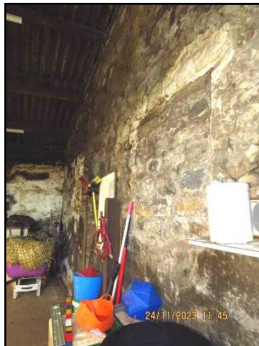
Photograph 054 Gable elevation looking to rear
