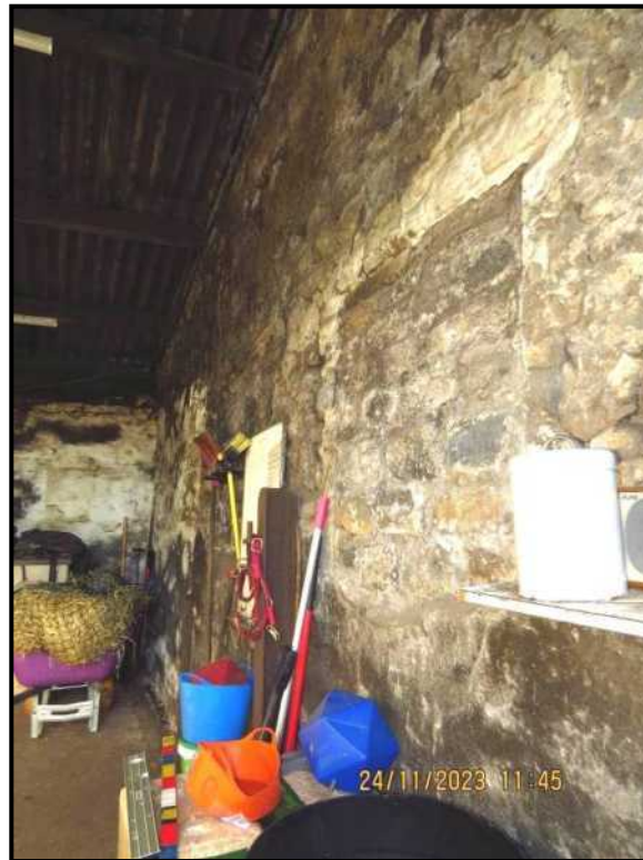
054 Gable elevation looking to rear
