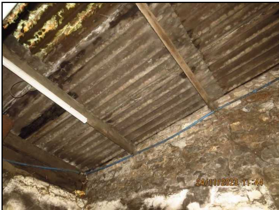
049 Eastern gable, roof support
