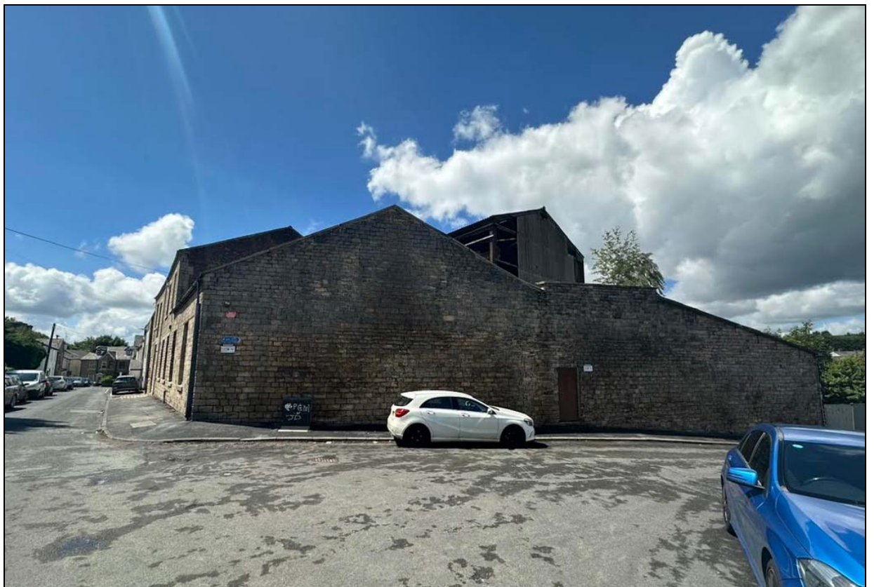
2. Wider view of the building from the New Street/Sweet Briar Lane junction
