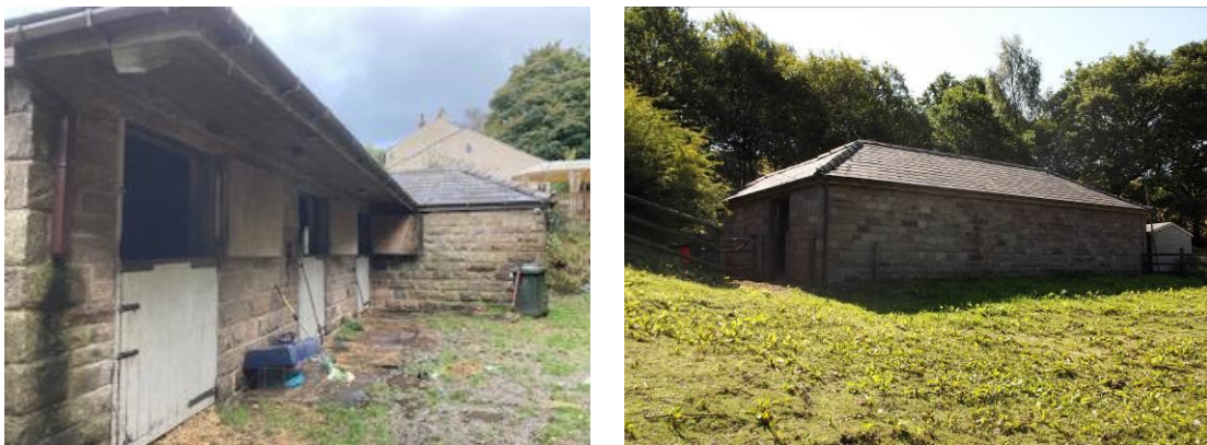
Plates 1 and 2. Front (south-eastern) and rear elevations
